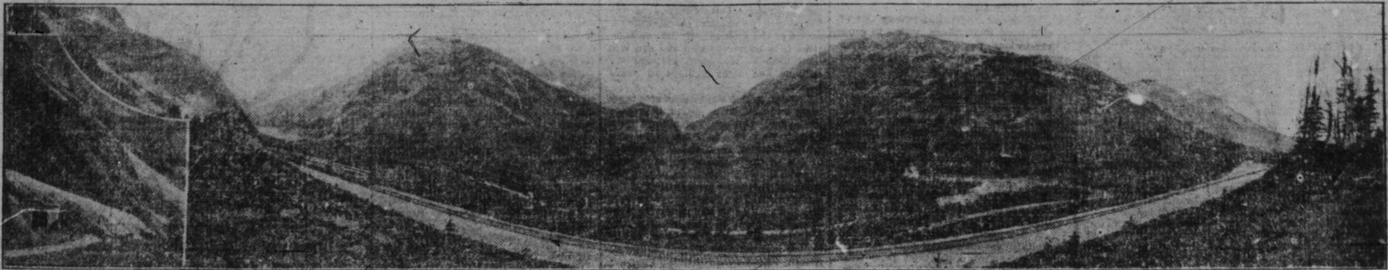
Entrance and outlet of Tunnel
