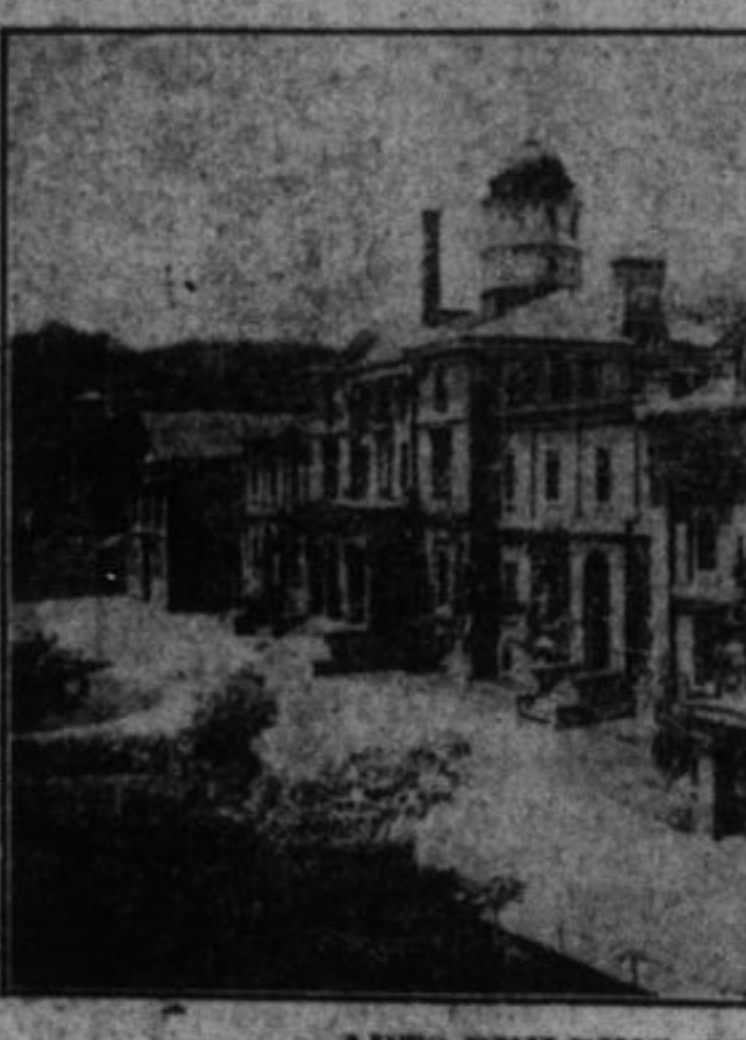
ARTS BUILDING, MCGILL COLLEGE.
