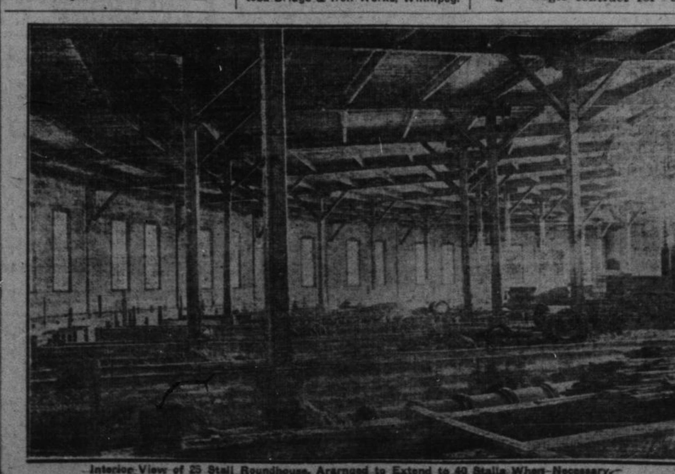
Interior View of 23 Steel Roundhouse, Arranged to Extend to 40 Stalls When Necessary.
