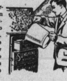
In the morning a gentle rocking of the lever removes all ashes from grates. No dust in operator's face, for he first opened damper into ust-pipe leading from ash-
