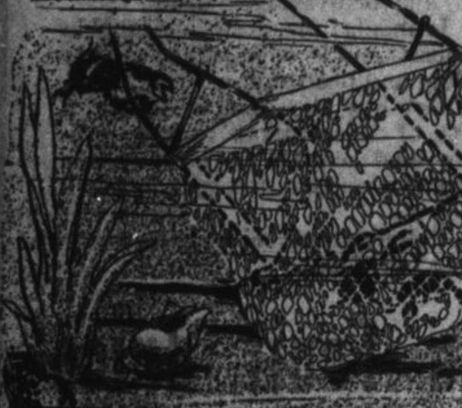
How the Dredge is Constructed
