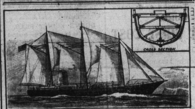
The ship now building in Mai ne for Commander Peary's next dash for the North Pole. It will be the strongest that has yet ventured into the ice fields; not only capable of forcing its way through frozen barriers, but of resisting enormous pressure. The latest ideas of construction, based upon experience with ice, are being employed by its builders. Pe ary hopes to put this vessel into winter quarters north of the eighty-second or eighty-third parallel.
