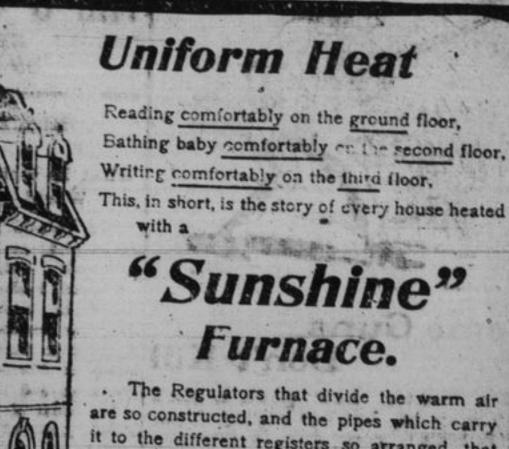
. The Regulators that divide the warm air are so constructed, and the pipes which carry it to the different registers so arranged, that any quantity of heat desired can be forced to the different rooms or flats of a house. The "Sunshine" is the only furnace made
