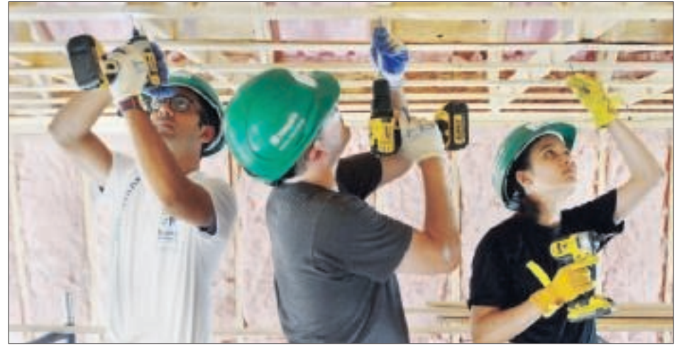
From left, Asad Nematullah, Frank Mercuri and Rebecca Archer install strapping.
