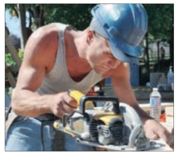
Tim Foster notches boards with a power saw.
