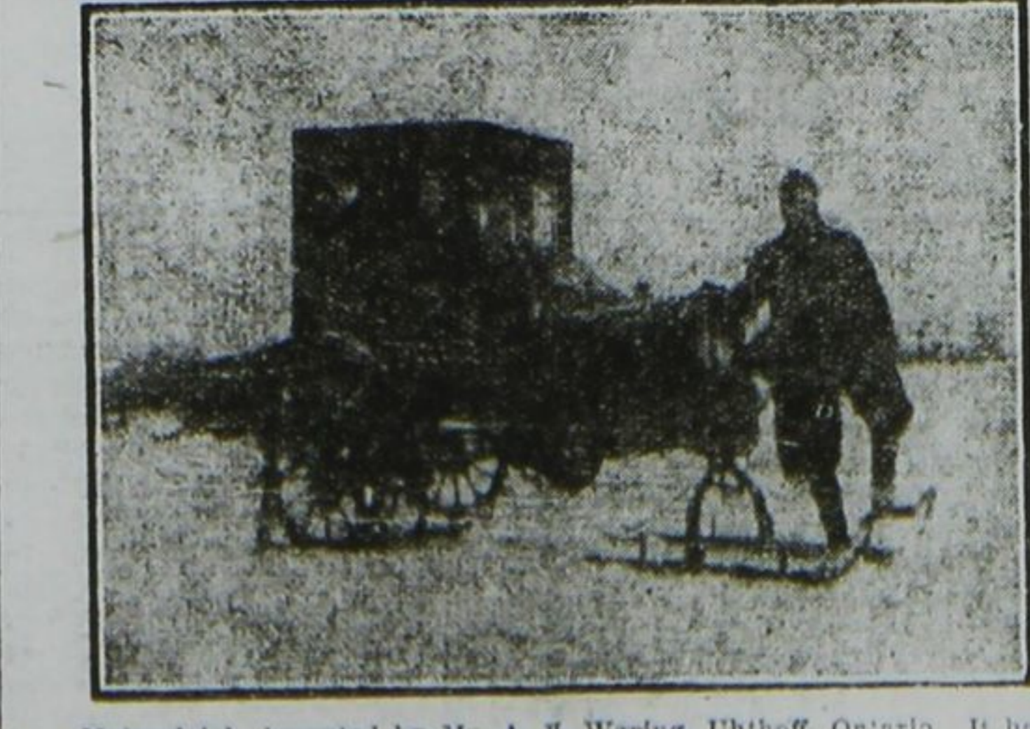
Motoreleigh, invented by Mr. A. H. Waring, Uthoff, Ontario. It has a Ford engine, and can travel twenty miles an hour on any road of ice or snow, and does not, like most motoreleighs, use excess gasoline.
