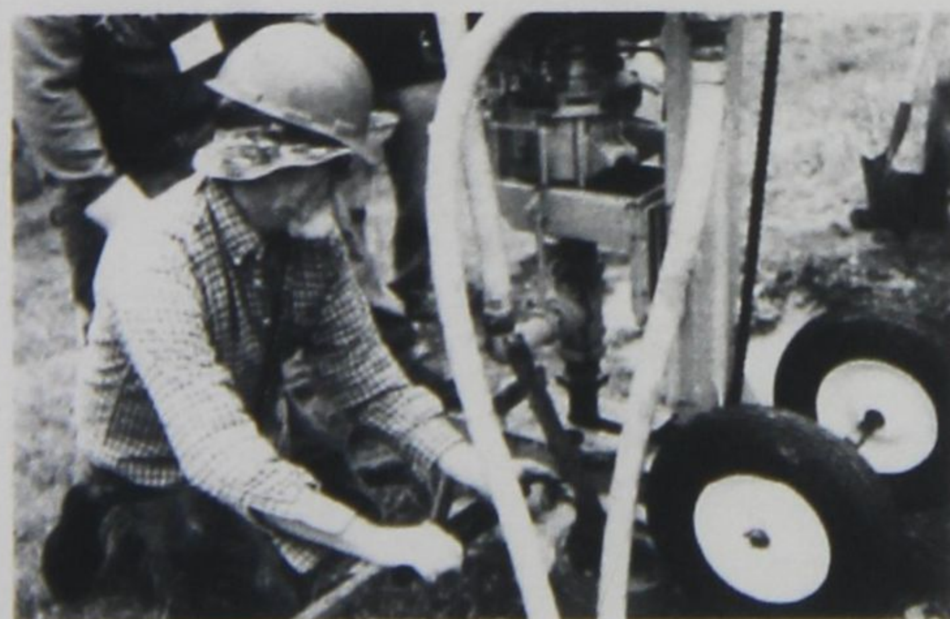
well drilling & repairs
