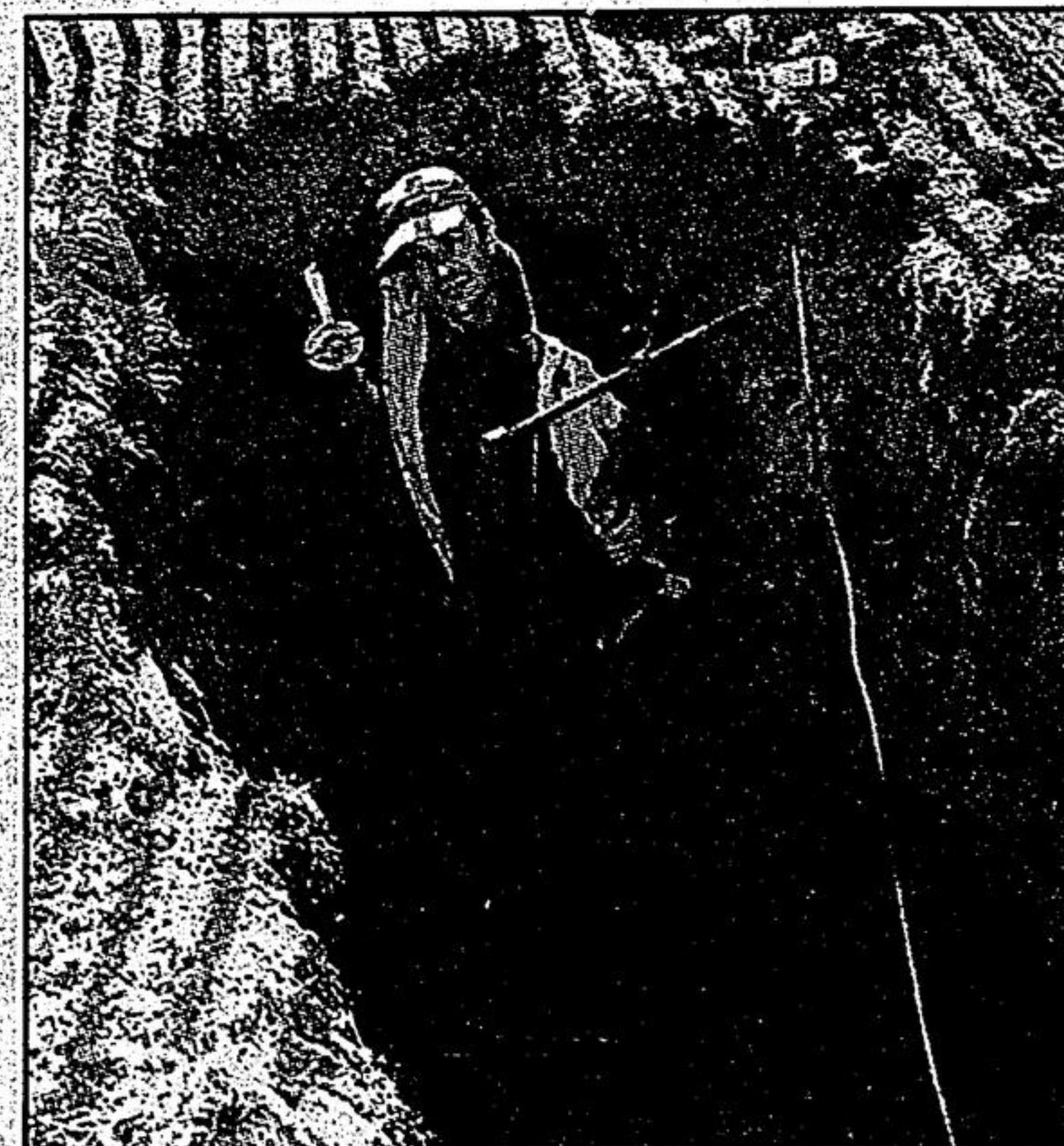
Mark Hassan, a plumbing contractor, is down about trenches he had to leave exposed over the weekend when regional plumbing inspectors refused to survey them.
