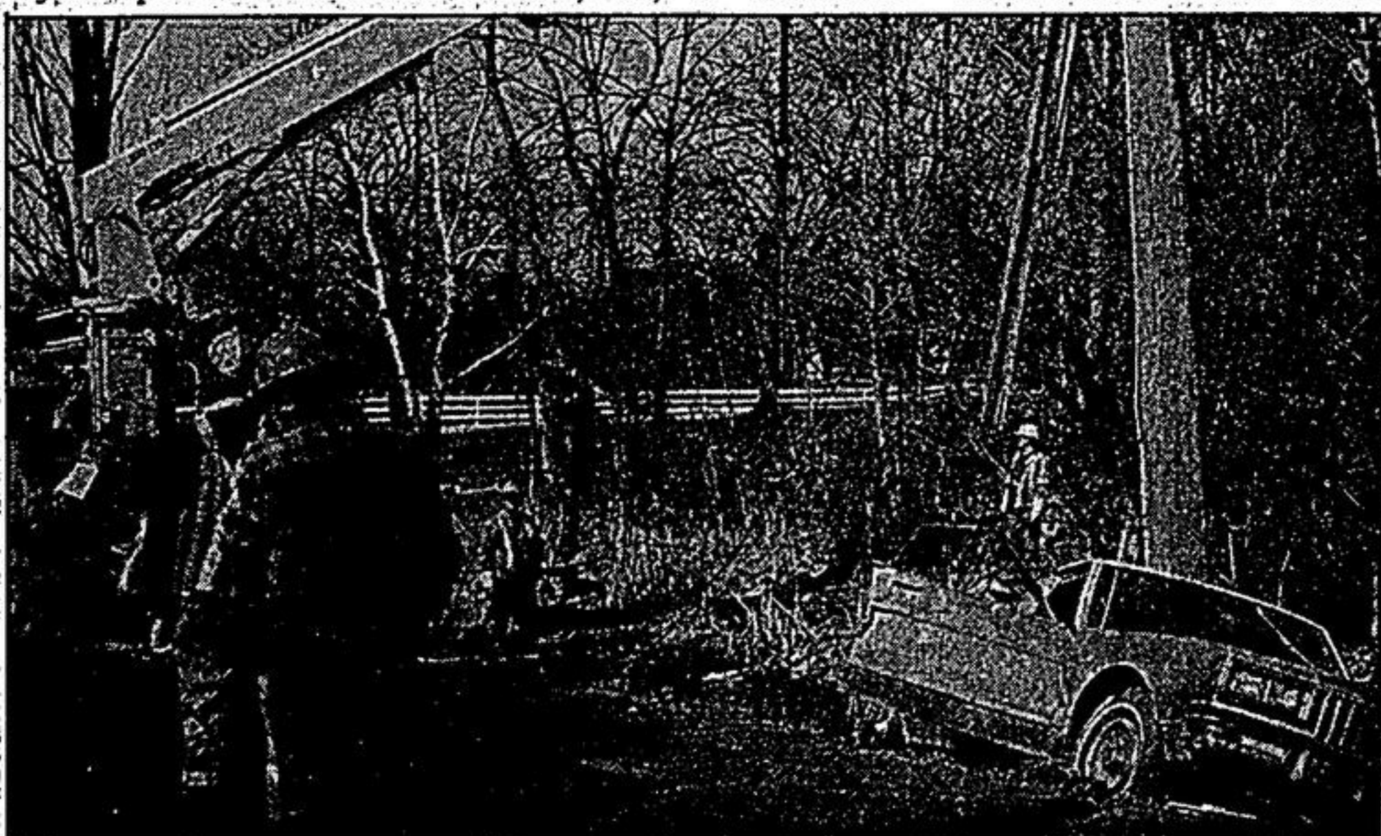
Hydro crews worked well into Monday afternoon to free this car so a new power line pole could be put in place after an accident that claimed the life of local florist James White on Sunday.
