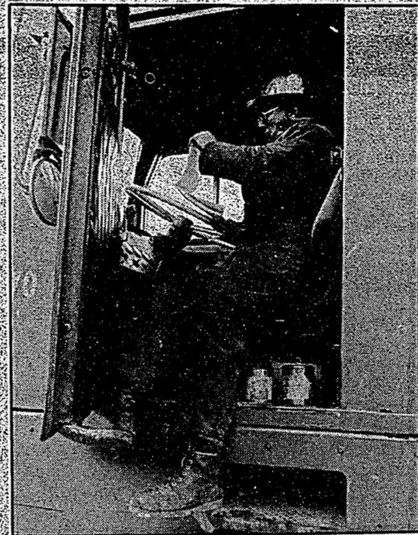
At left, Eric Benns, top left, watches the crew attach the third beam. Below, crane operator Allan Wilson checks his paperwork. The bridge reinforcements were completed before Christmas. Finishing will take place in the new year.
