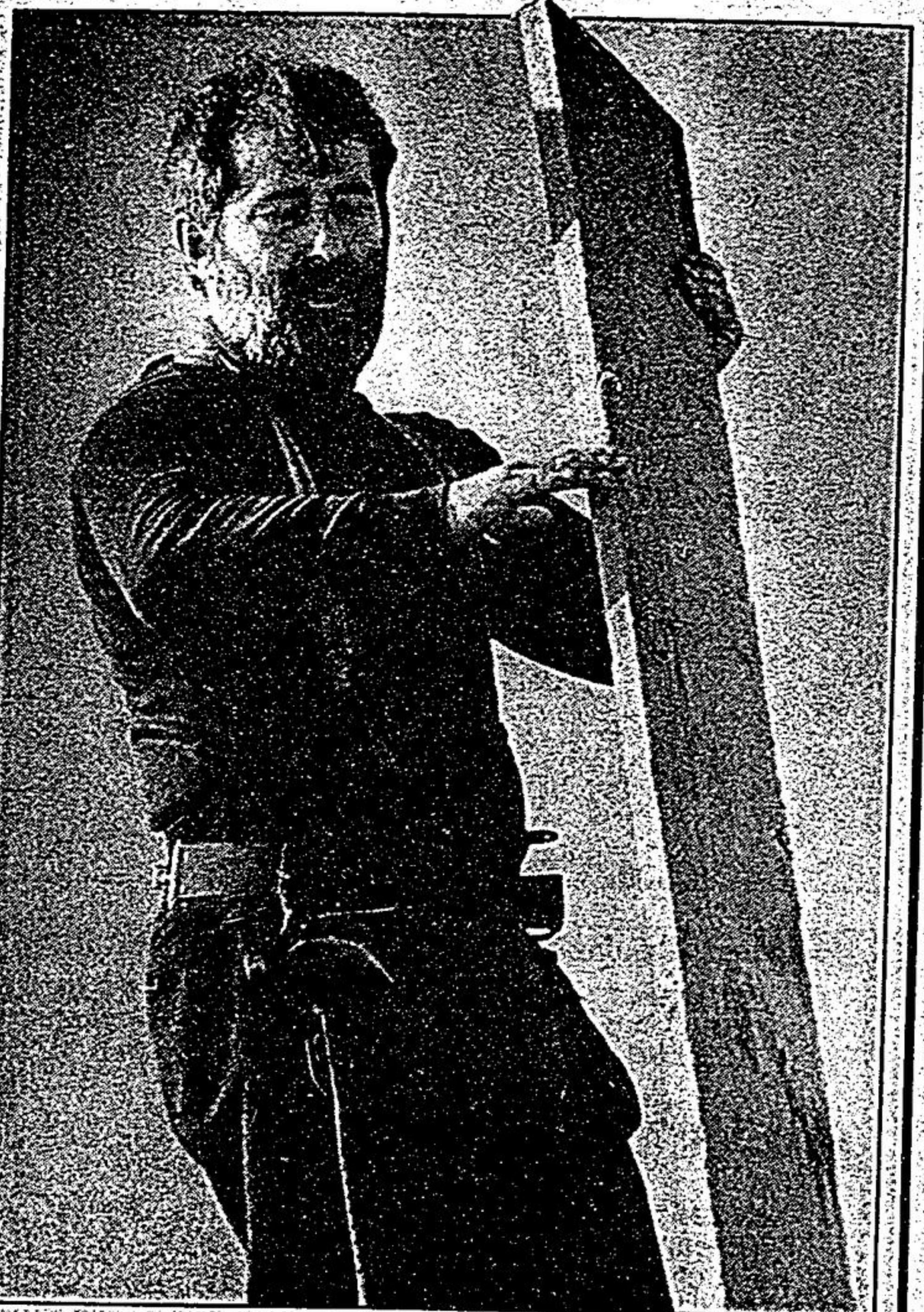
Jack Gubser checks the length of roof board.
