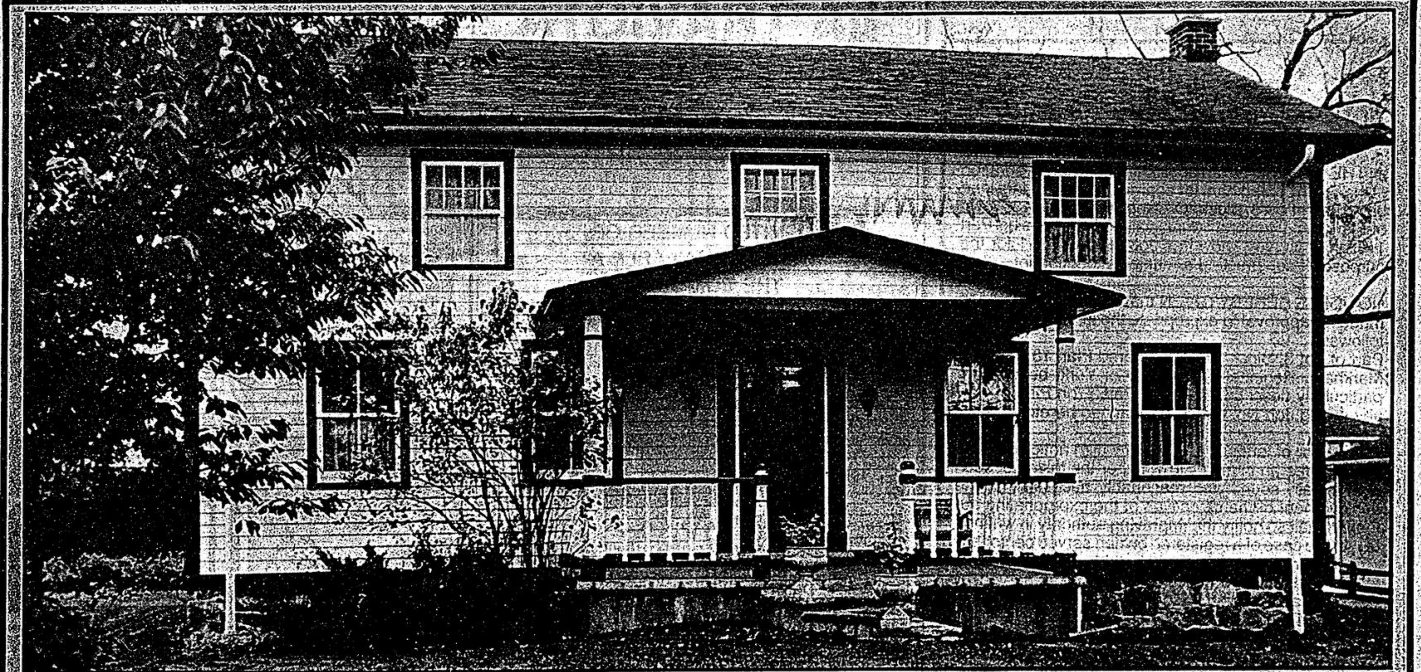
This fully restored farm house features a hand carved mantel on the living room fireplace. It is listed for $285,000.
