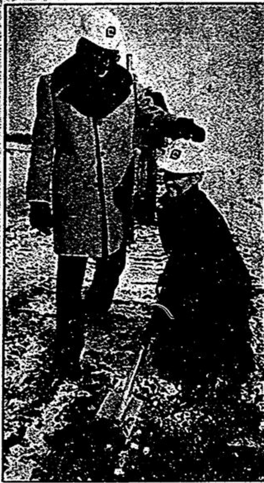
Markham Mayor Carole Bell (right) and Frank Holmes, vice president of administration and finance for Semi-Tech Microelectronics Corporation, break ground for the new research and development plant at Steeles and Warden avenues last week.
