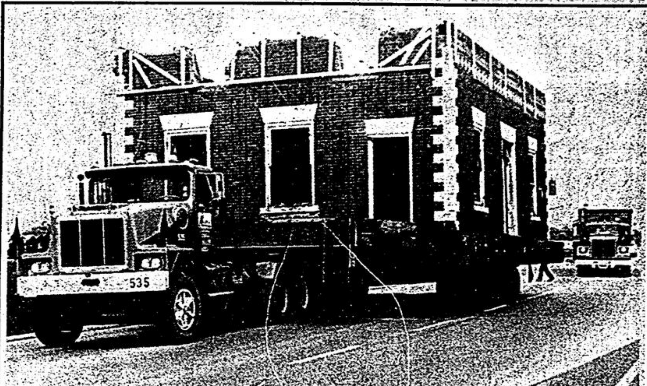
Historic Stouffville house finds a new home The Brown family house, believed to be more than 120 years old, has found a new home. Last week, it was moved by Anderson Haulage from a site, north of the Stouffville Sales Barn to the Whitchurch-Stouffville Museum at Vandorf. The late Wm. Brown, an original owner, is the great-great grandfather of Ross Brown, Montreal Street and Marie Jack, Second Street, Stouffville. —Jim Holt
