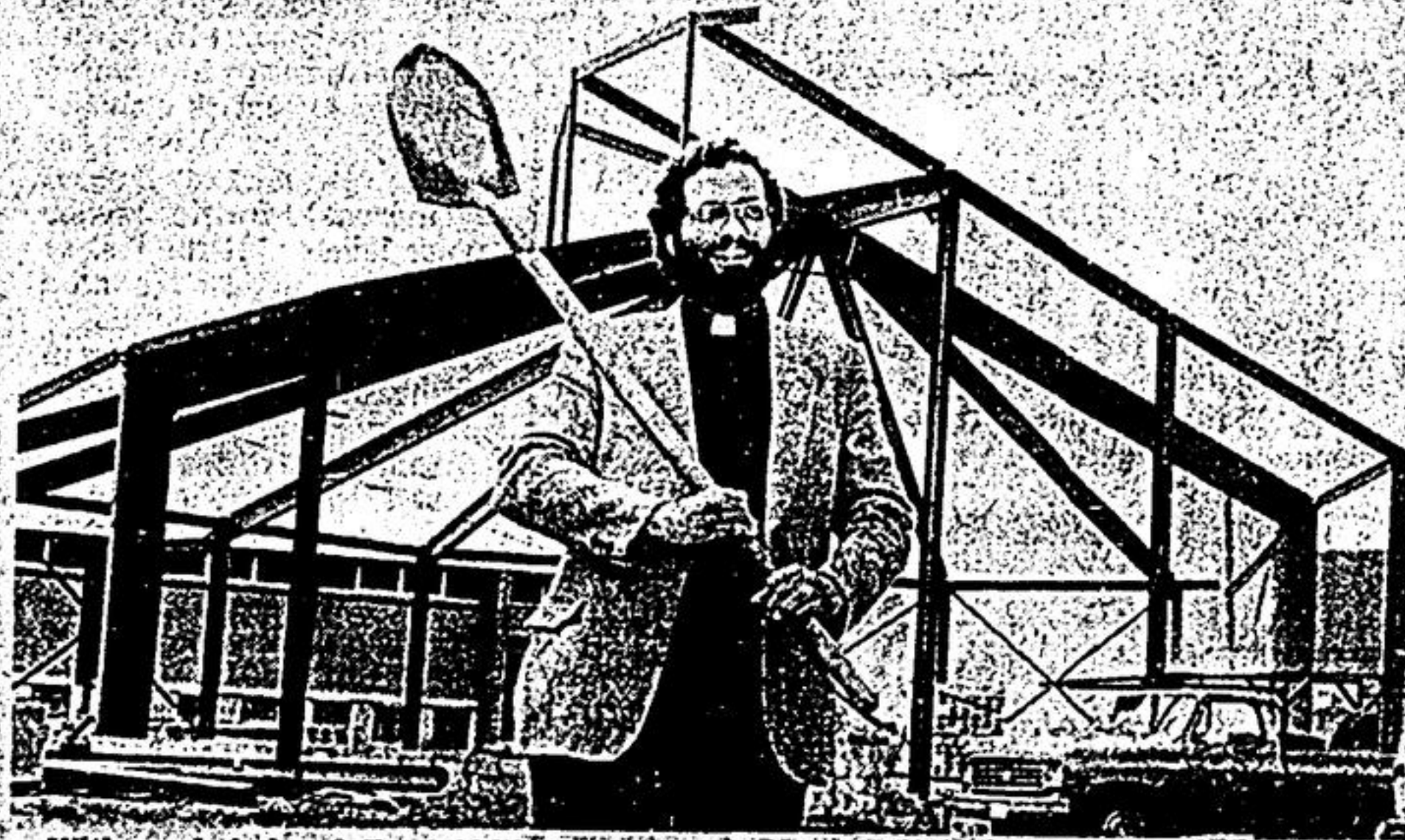
With spade in hand, Rev. Philip Poole of Christ Church (Anglican), Stouffville, contemplates his next odd job as construction work goes on behind him. Target date for completion of the $380,000 project is mid-October.
