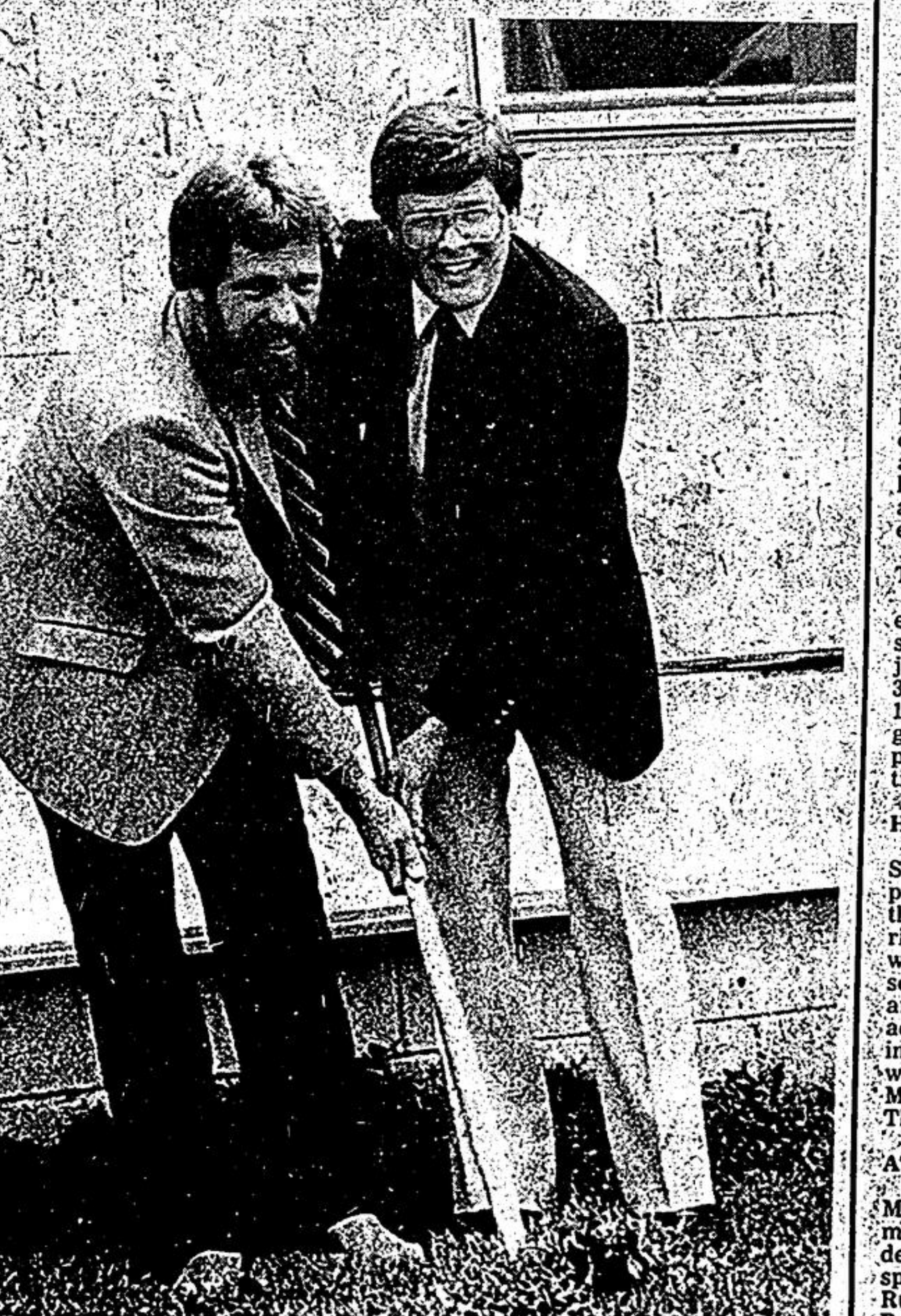
Addition to Springvale Baptist Church A major addition is planned for Springvale Baptist Church at the corner of Kennedy Road and the Stouffville Road in Whitchurch-Stouffville. To mark the project's beginning, a sod-turning ceremony was held Sunday with Rev. Robert Flemming, (right), and Phil Hutchinson taking part. The addition will include a full sanctuary to seat more than 400. Cost of the project is estimated at $400,000 with construction scheduled to start July 3. -Chris Shanahan
