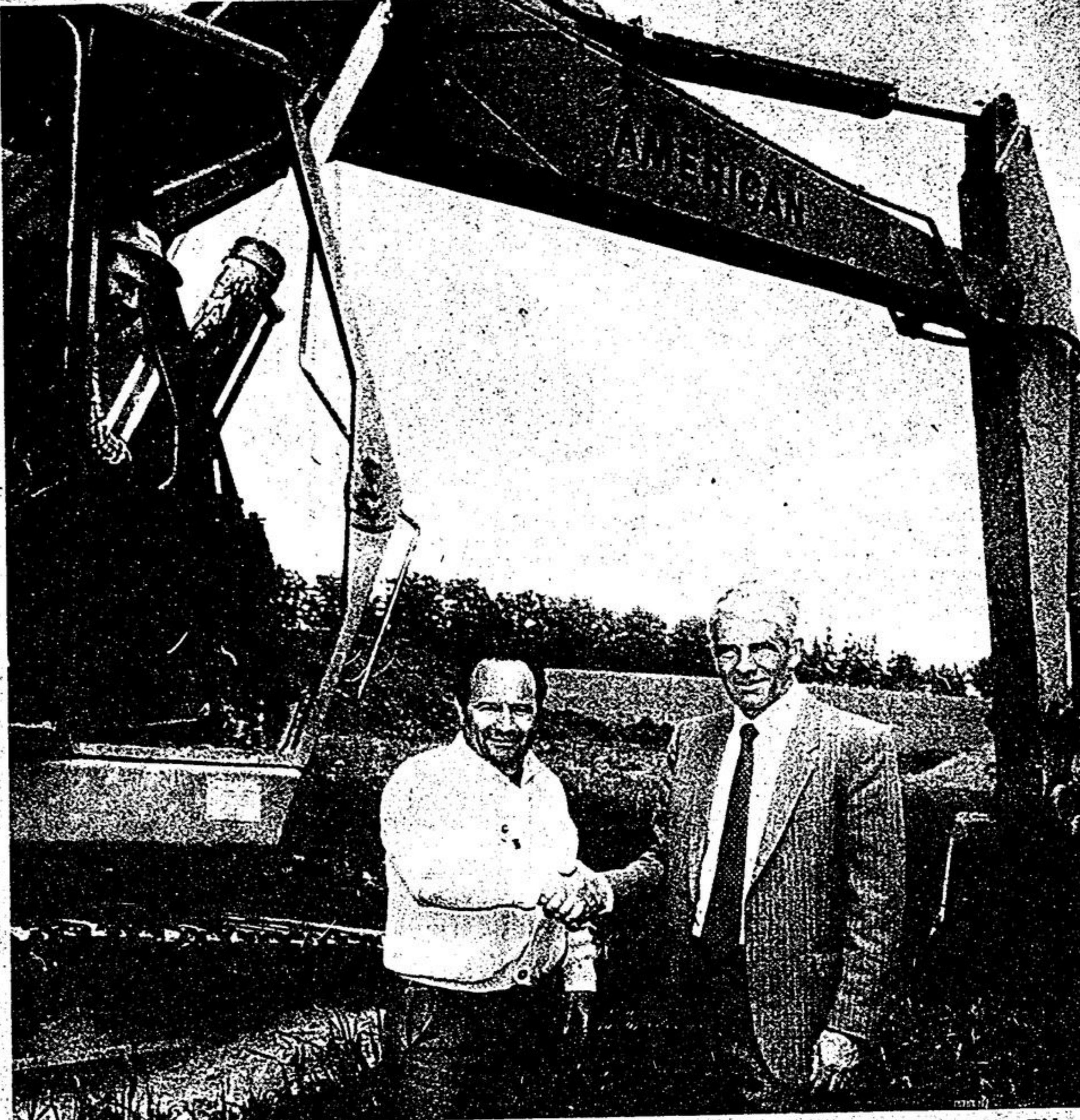
Construction commenced Friday at the site of the long-awaited Dulverton Development in Stouffville. Five model homes will be built "to test the market". If these are enthusiastically received, 100 more will follow. In attendance at an informal ground-breaking ceremony was Mayor Eldred King; builder Frank Mauro and back-hoe operator Peter DelMastro. The subdivision agreement calls for a total of 576 residences when completed. —Jim Thomas
