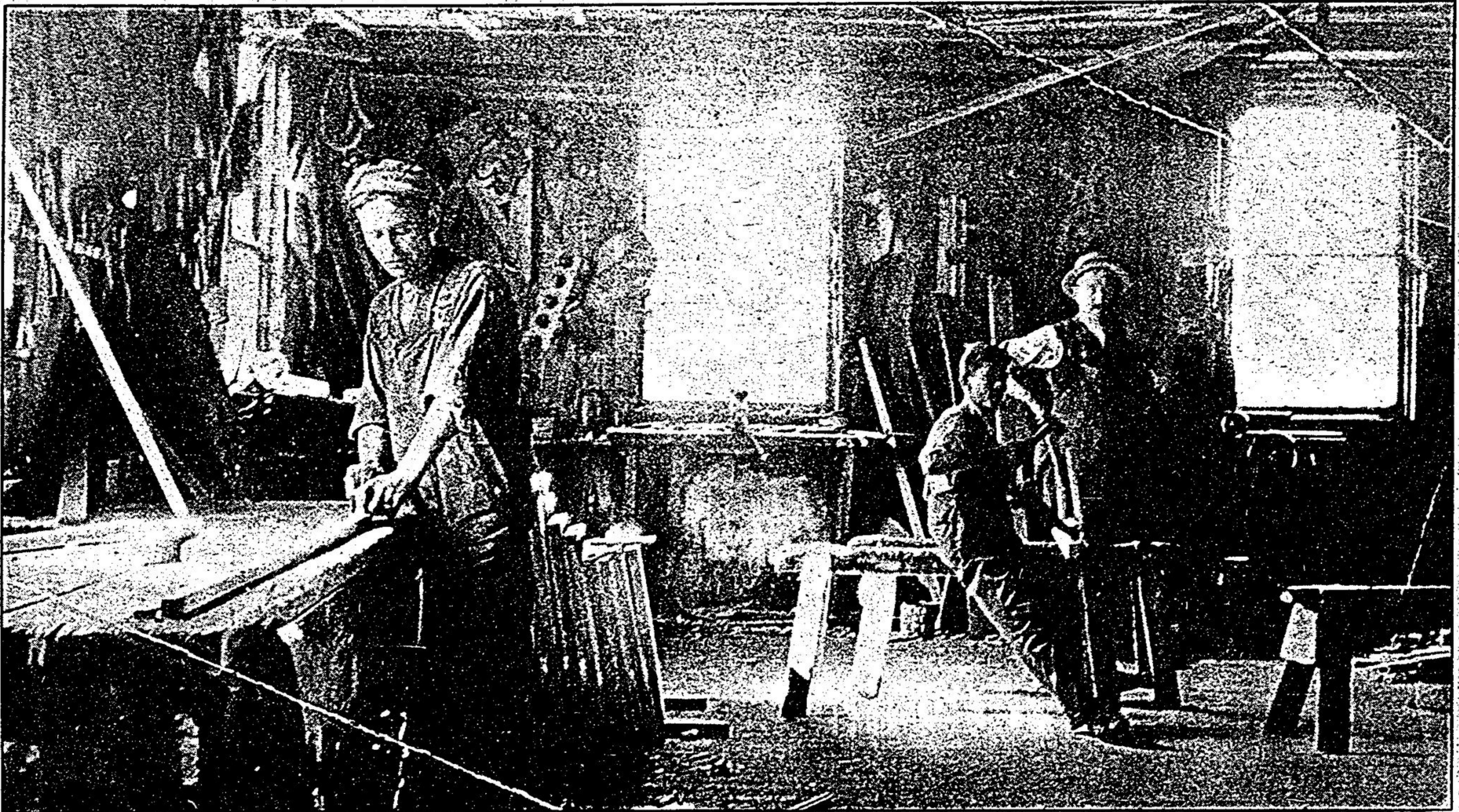
Rare photo of the upstairs workshop interior of the Unionville Planing Mill recently lost to fire. On far right is De Harrington, proprietor. See feature story Page 9.
