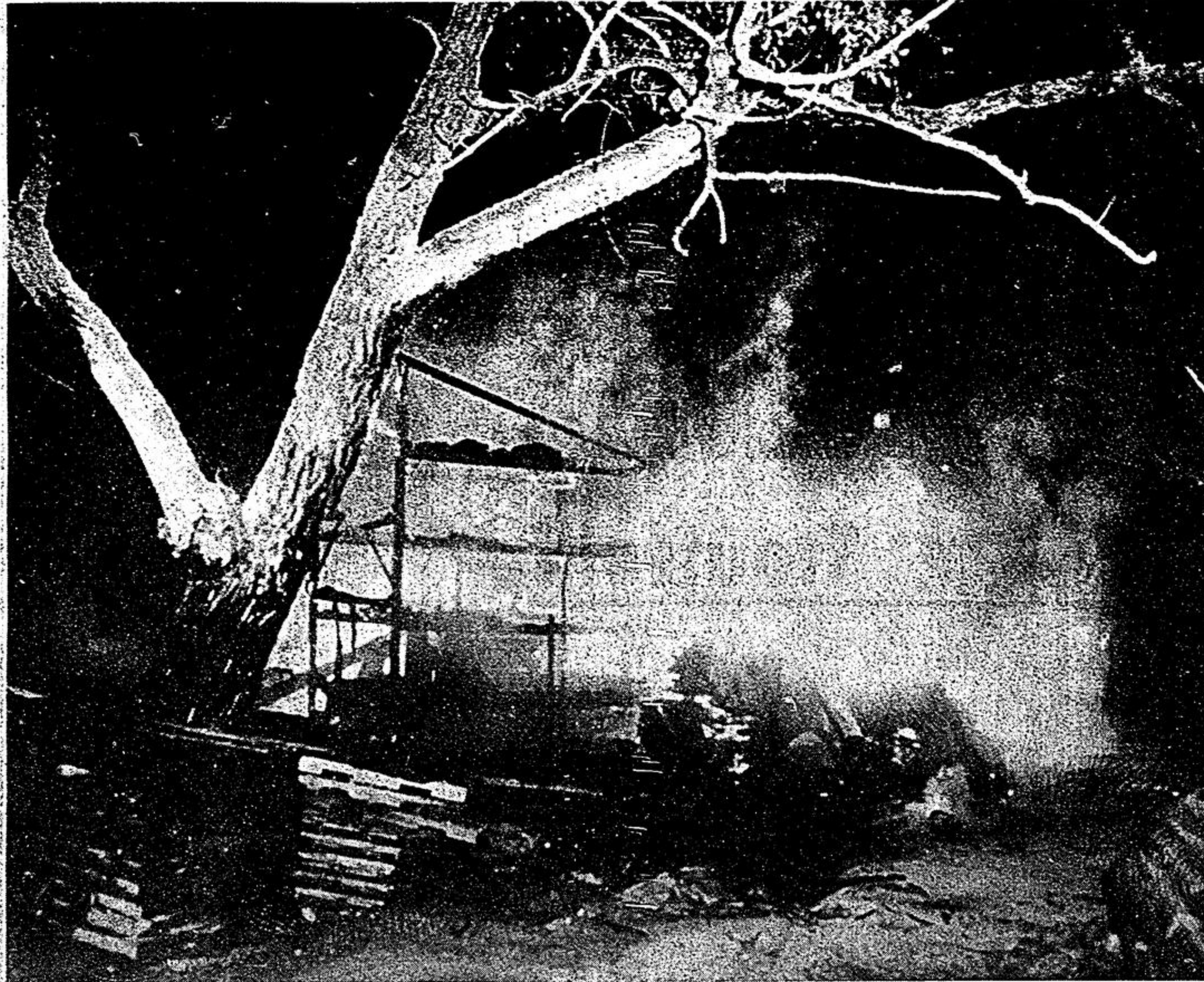
Fire attributed to lightning, destroyed a 130 year old sawmill, Friday morning at Century Mill Industrial Lumber, R.R. 4, Stouffville. Property damage, including 35,000 board feet of
