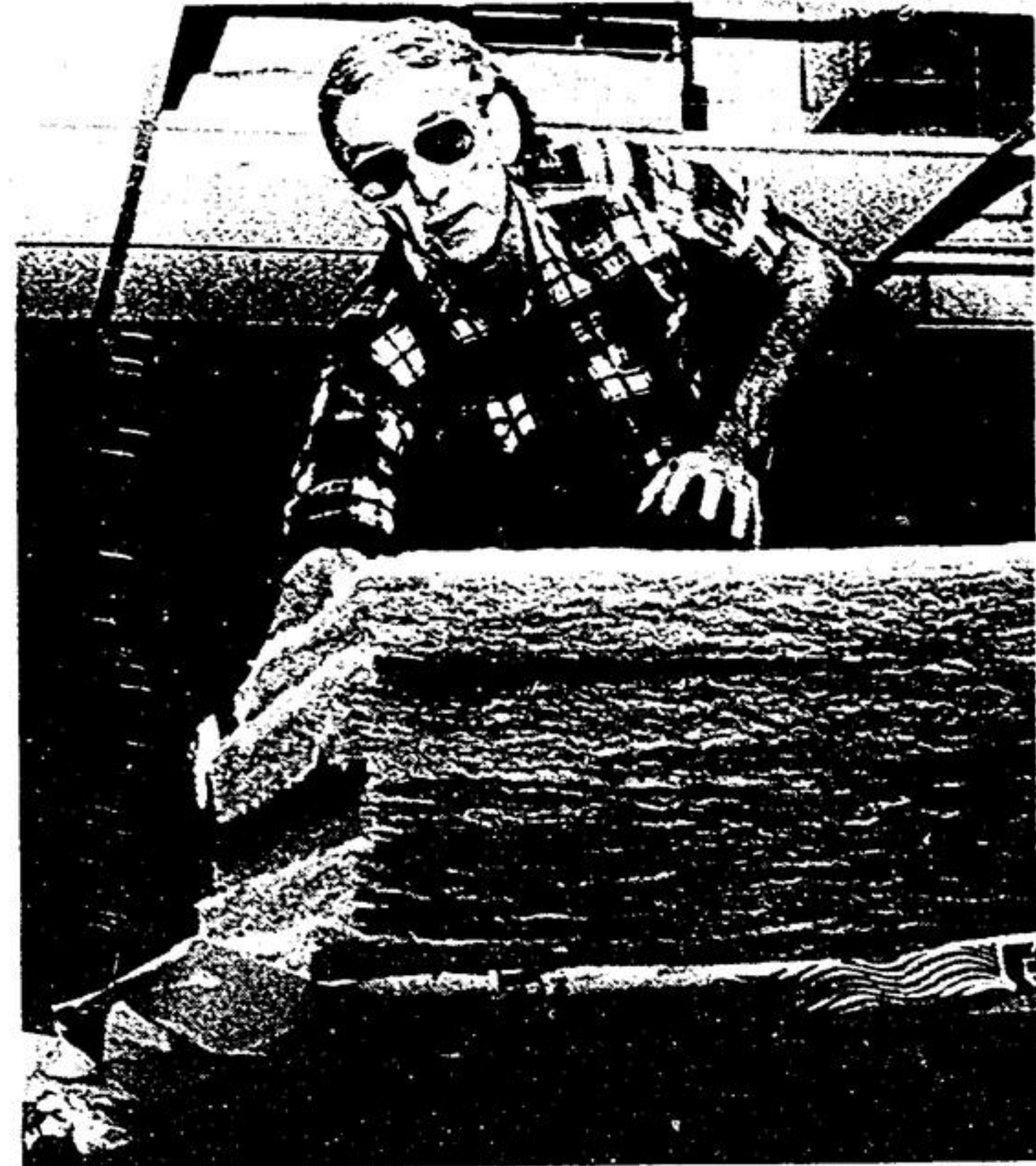
Kim Rogers of Ballantrae was a driving force behind a do-it-yourself project, recently, that installed insulation in the Community Centre there. The Town supplied the materials but all the work was volunteer.
