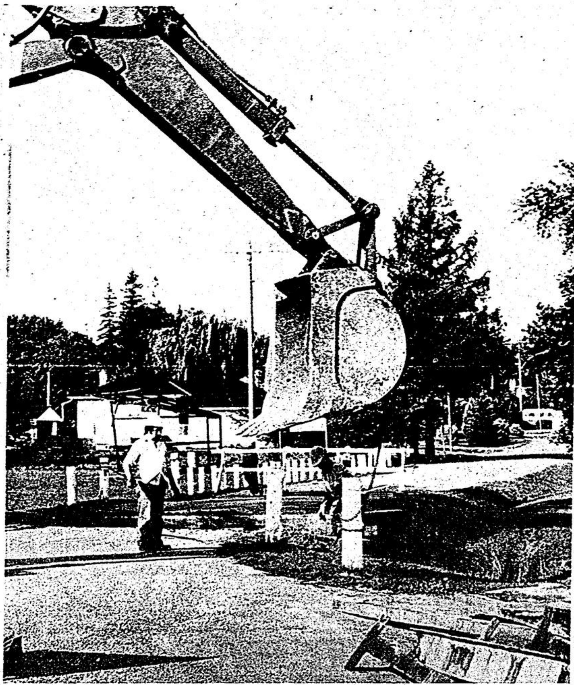
Begin long-awaited channelization project
