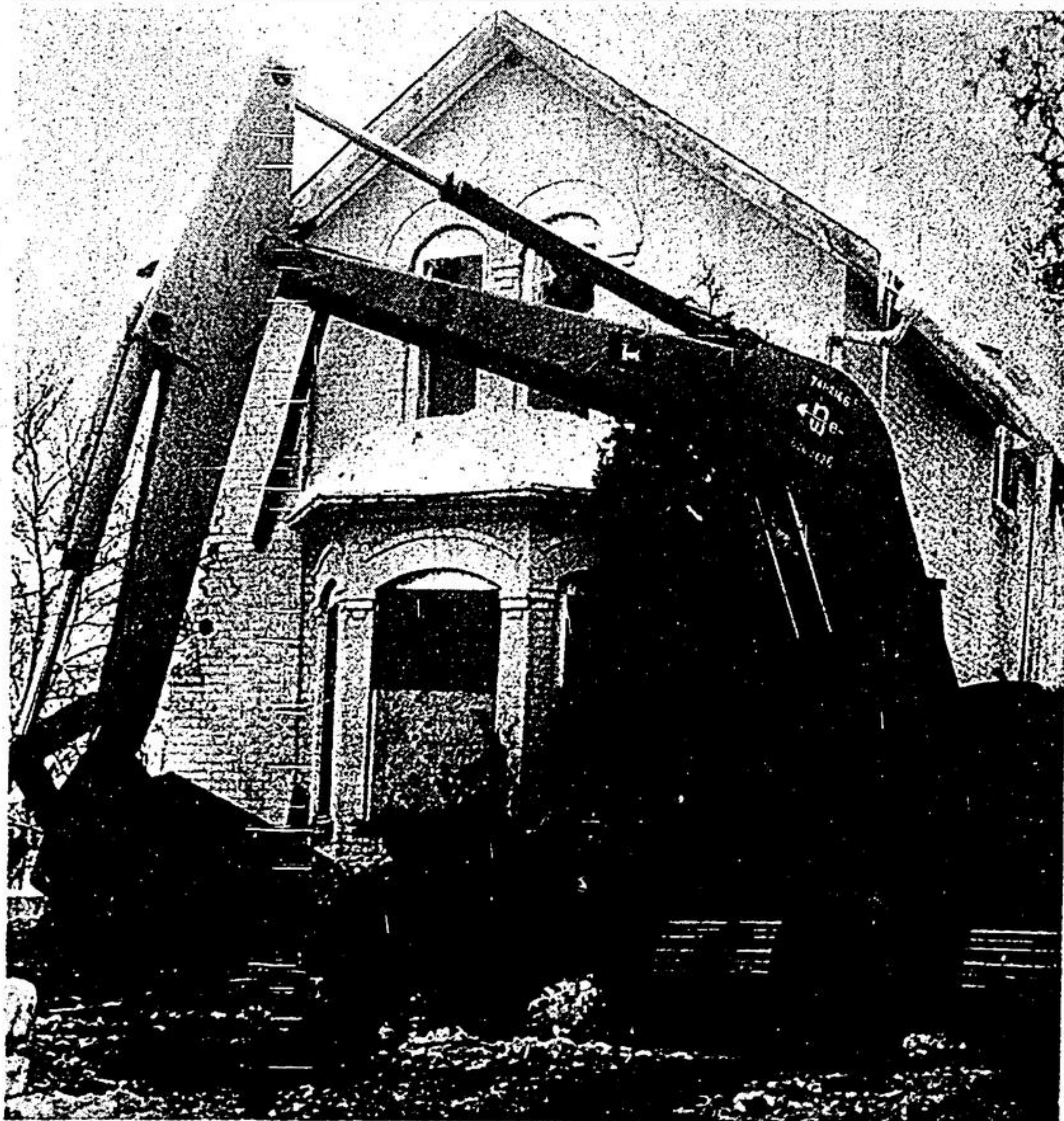
"Progress" levels another Town landmark
