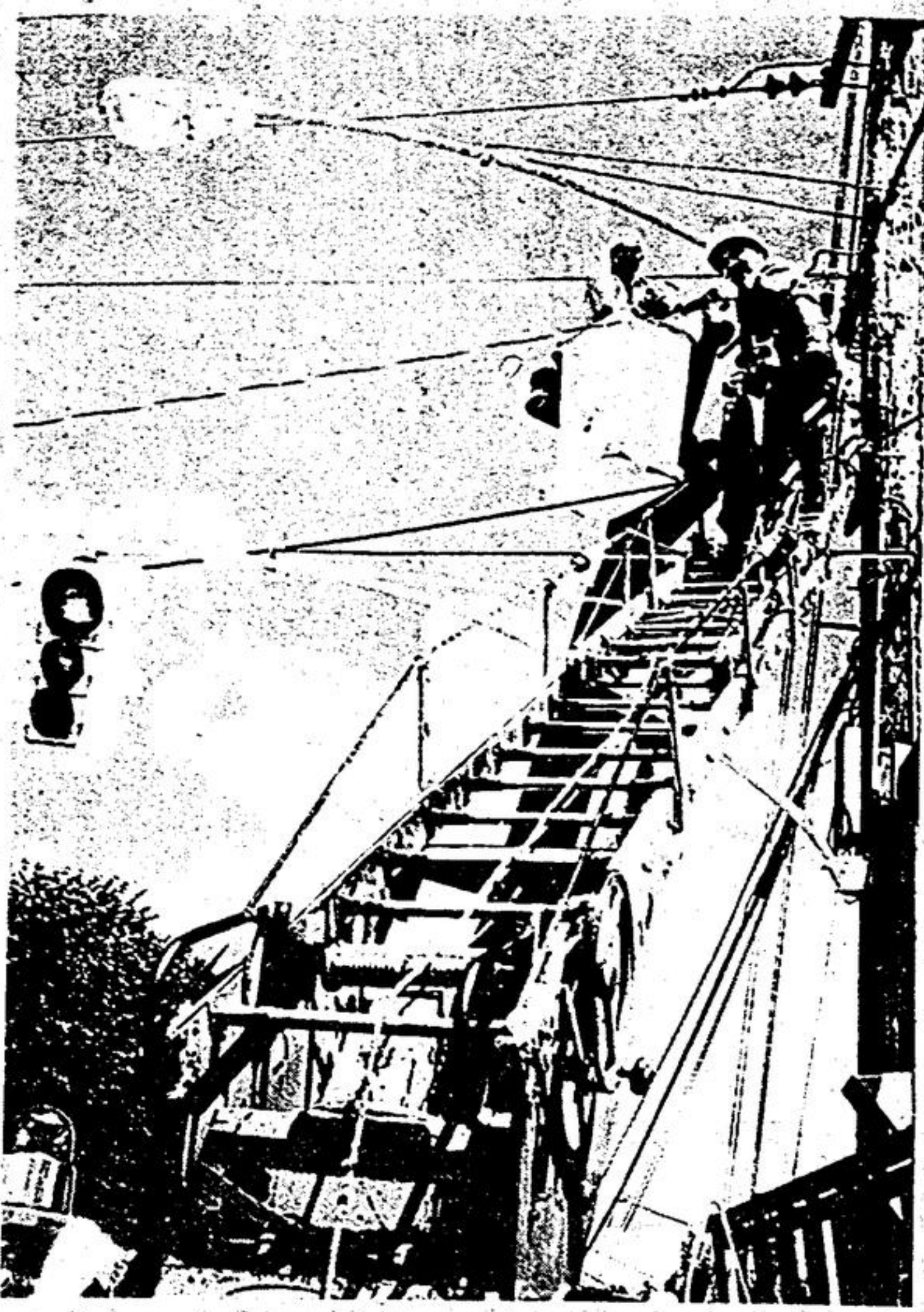
Visibility should be much improved at the intersection of Main St. and the 9th line following installation of these modern street lamps. Here Charles Lintner (in basket) and Carl Wideman are completing the hook-up.
