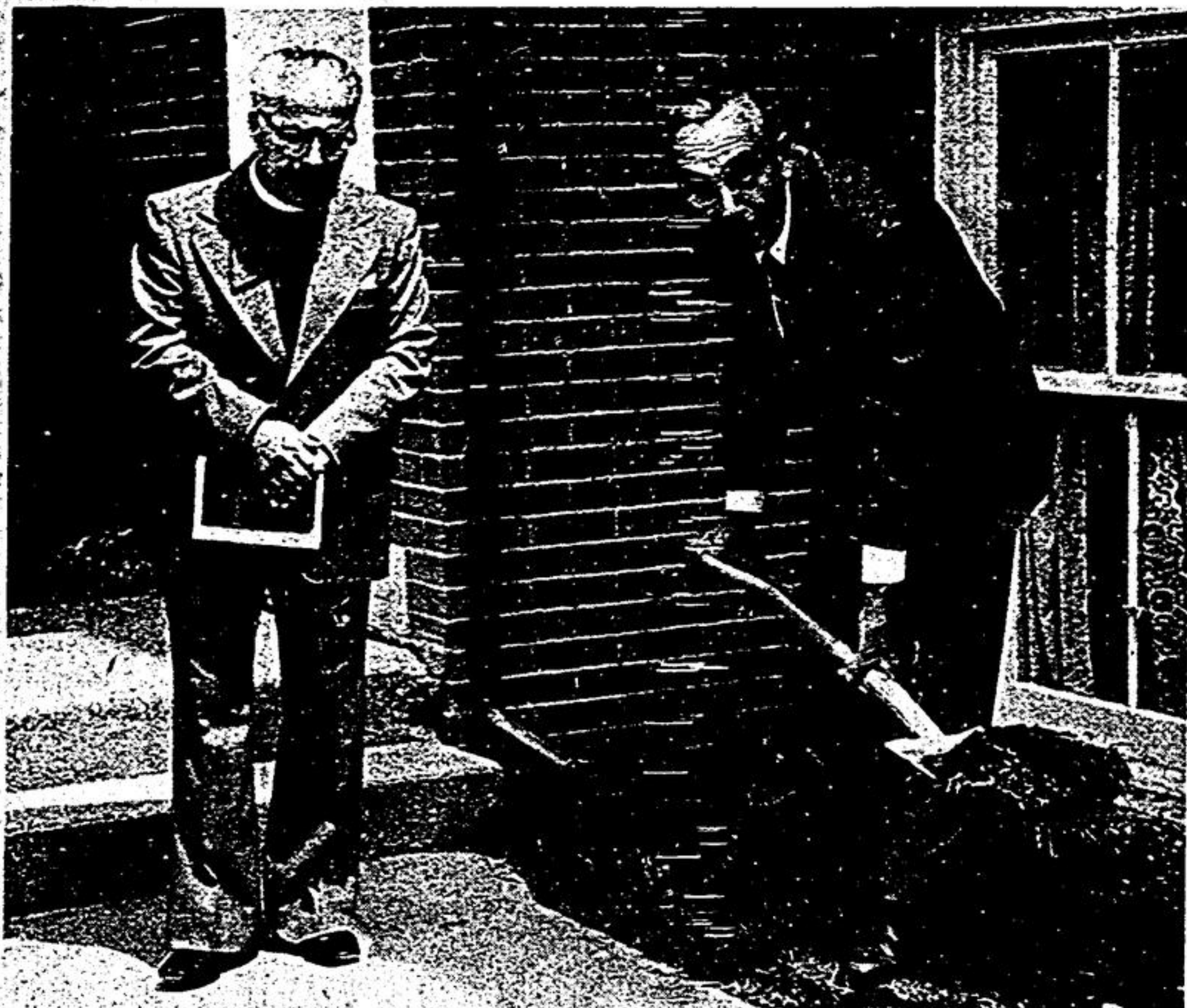
United Church Congregation held a sod turning ceremony following the service Sunday. The new addition, which is expected to cost about $130,000, will include Sunday School rooms, minister's study, a library and a new entrance at the south west corner which will include an electric chair lift for those unable to climb stairs. Secretary of the Congregational Board Charles James is shown here turning the sod while Rev. J. L. Carder looks on. A short open air service was conducted.
