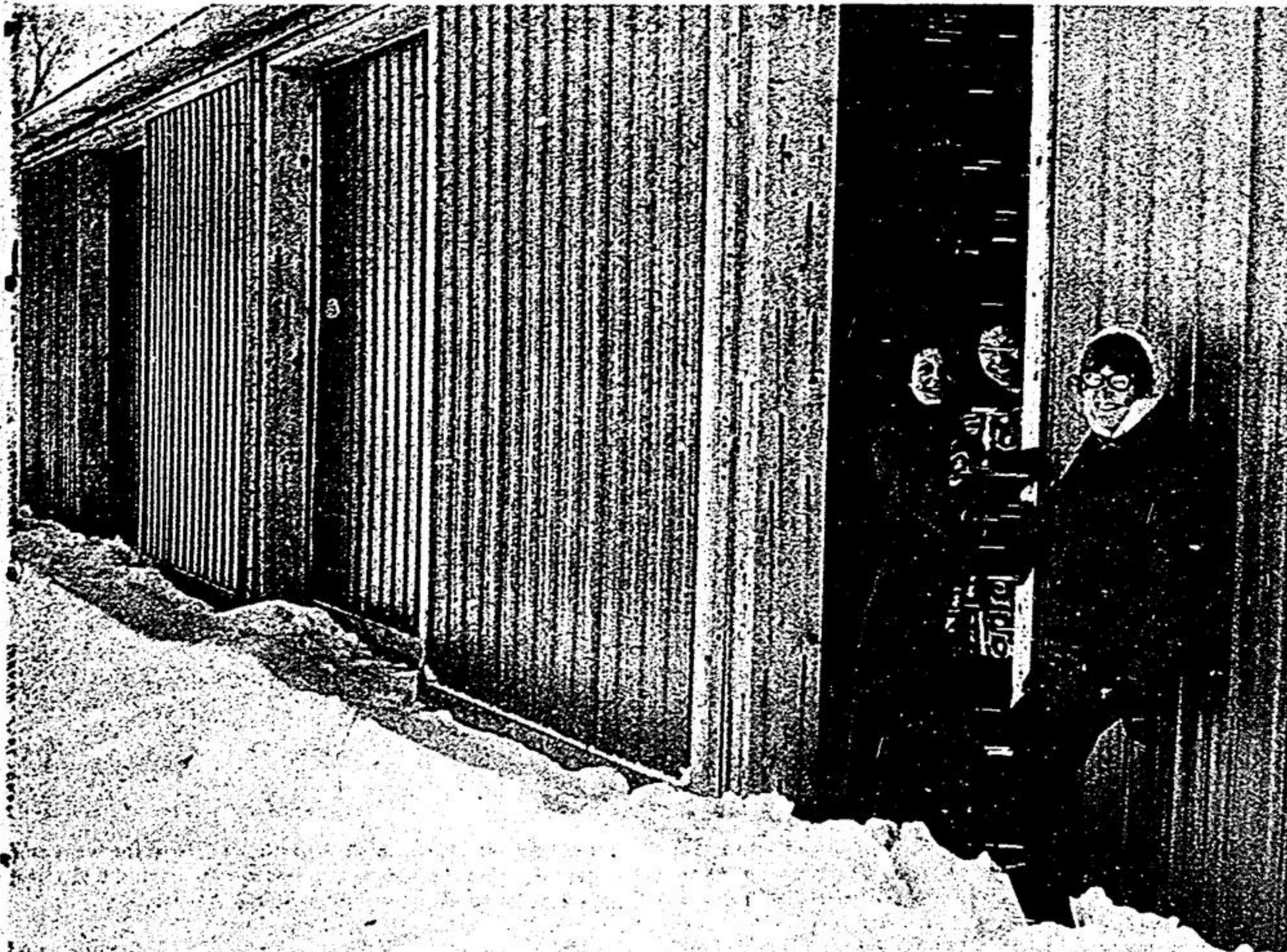
Saturday morning is the official opening of Stouffville's new recycling depot. Here, three of the ladies who work at the depot try out the newly installed sliding doors. The new building, which will be shared with the town Works Department, will allow the refuse bins to be stored inside. Mayor Gordon Ratcliff will be on hand Saturday morning at 11 a.m. for the official opening. The depot now serves about 500 families in Whitchurch-Stouffville. Shown here are Mable Smith, Jean Bellisle and Joice Nailer. —Don Bernard
