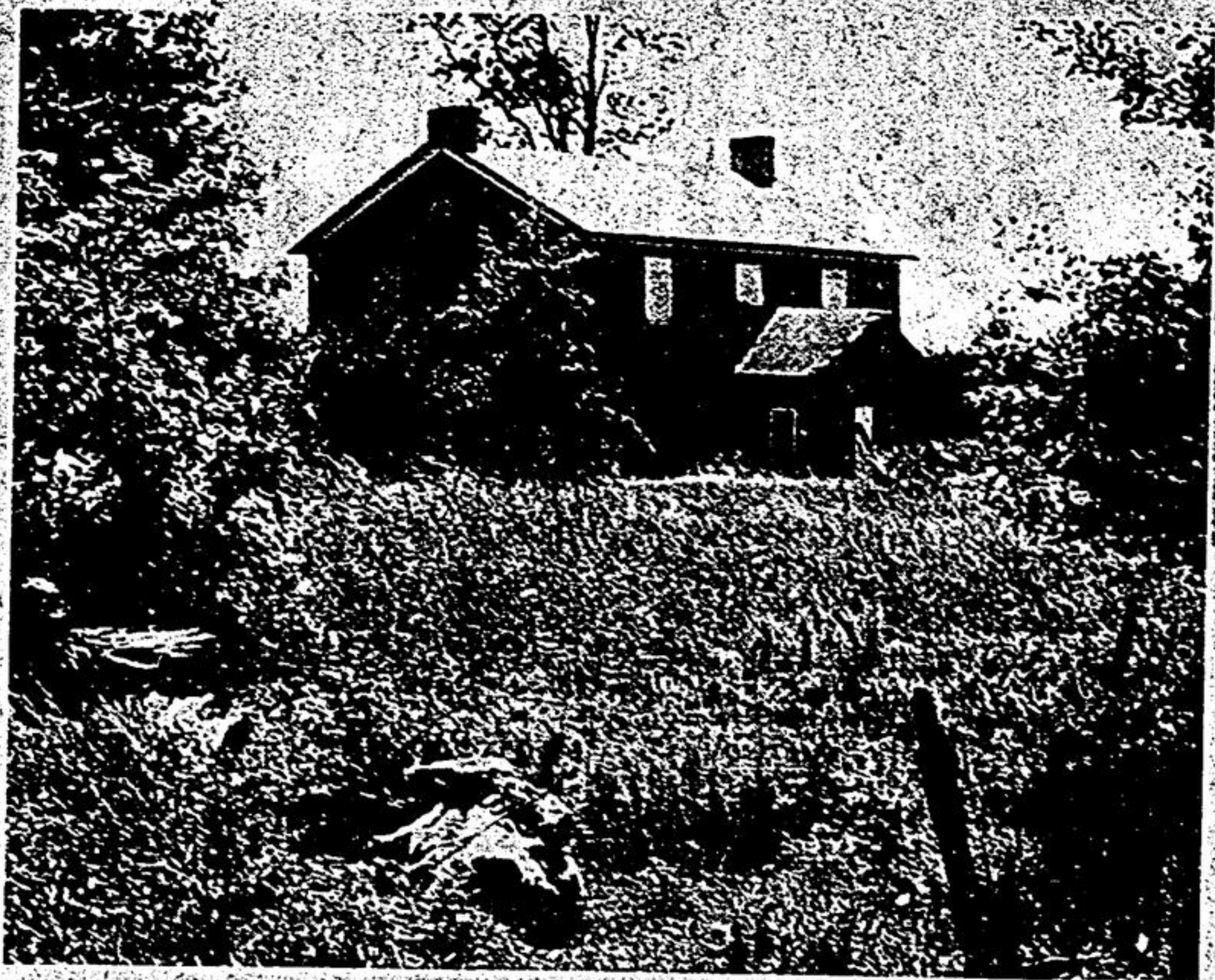
Boarded up houses, many now being demolished for the Pickering airport, are mute testimony to the sad spectre of century houses reduced to rubble by bulldozers. This one is located on Sideline 24, south of the 8th Conc. —Don Bernard
