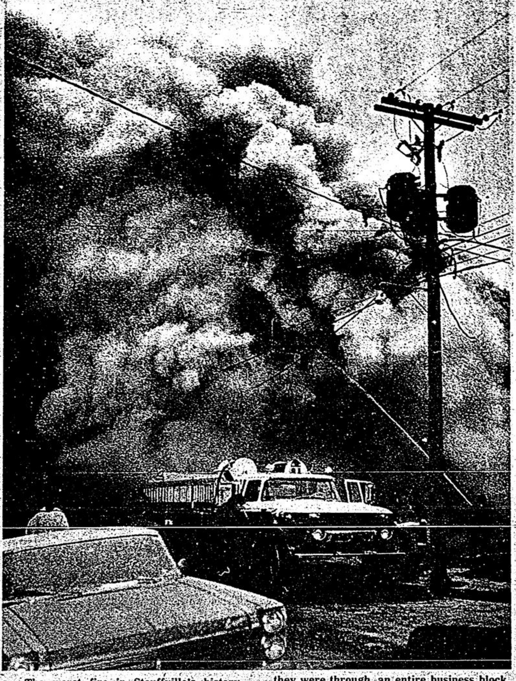
The worst fire in Stouffville's history destroyed the Ratcliff block on Nov. 11, 1971. The blaze was discovered around 8 a.m. in the morning. It took 60 volunteers from five fire brigades, 34 hours to extinguish the fire. When they were through, an entire business block, including eight second and third storey apartments, were destroyed.
