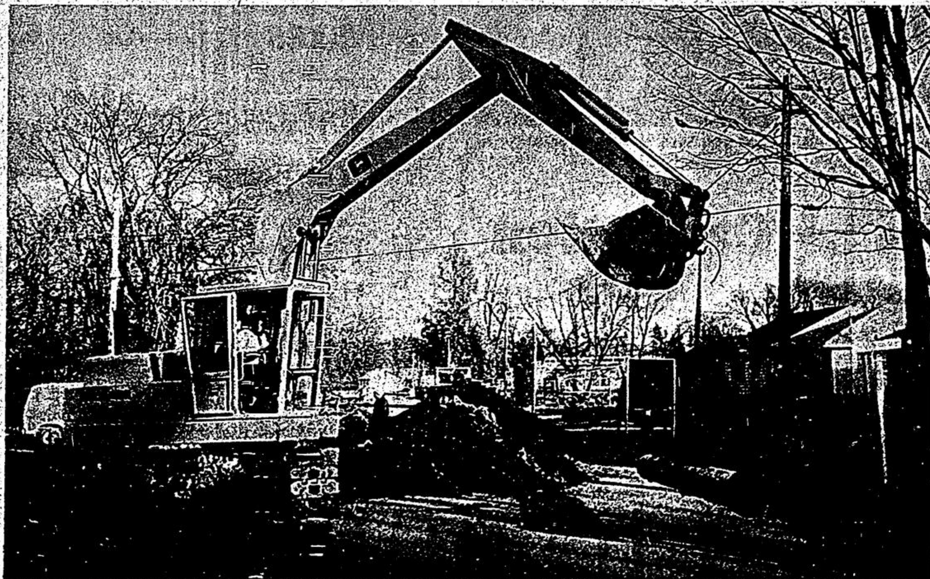
First phase of cross-town water main soon completed
