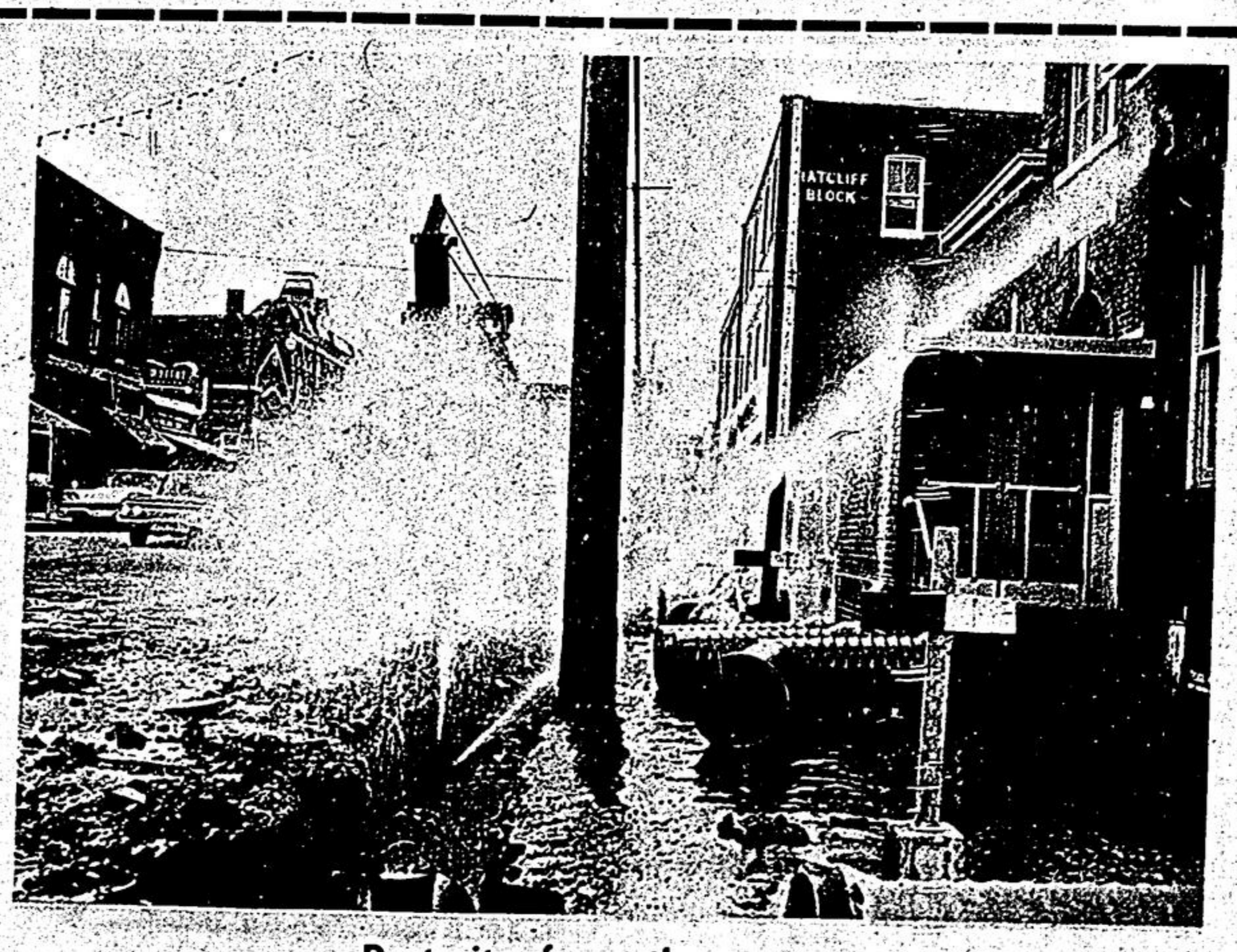
Portraits from the past Remember this geyser on Main Street? It occurred in November, 1960 in front of the Stouffville Post Office when a power shovel snapped a water pipe under 60 pounds of pressure. —Jas. Thomas
