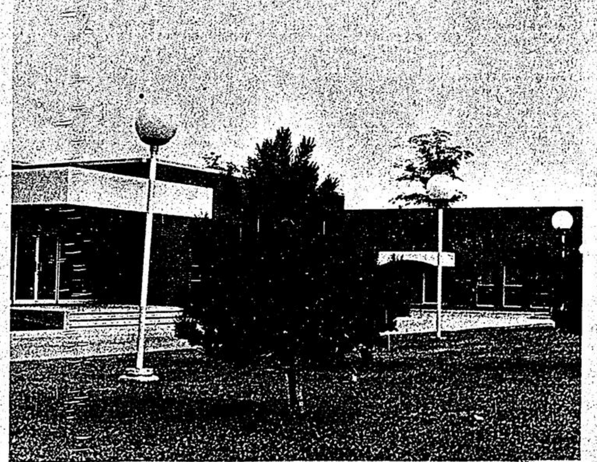
Wrentham Court located on Leslie St. in Metropolitan Toronto is a multiple tenancy building, with office area fronting the court and warehouse and loading platforms at the rear.
