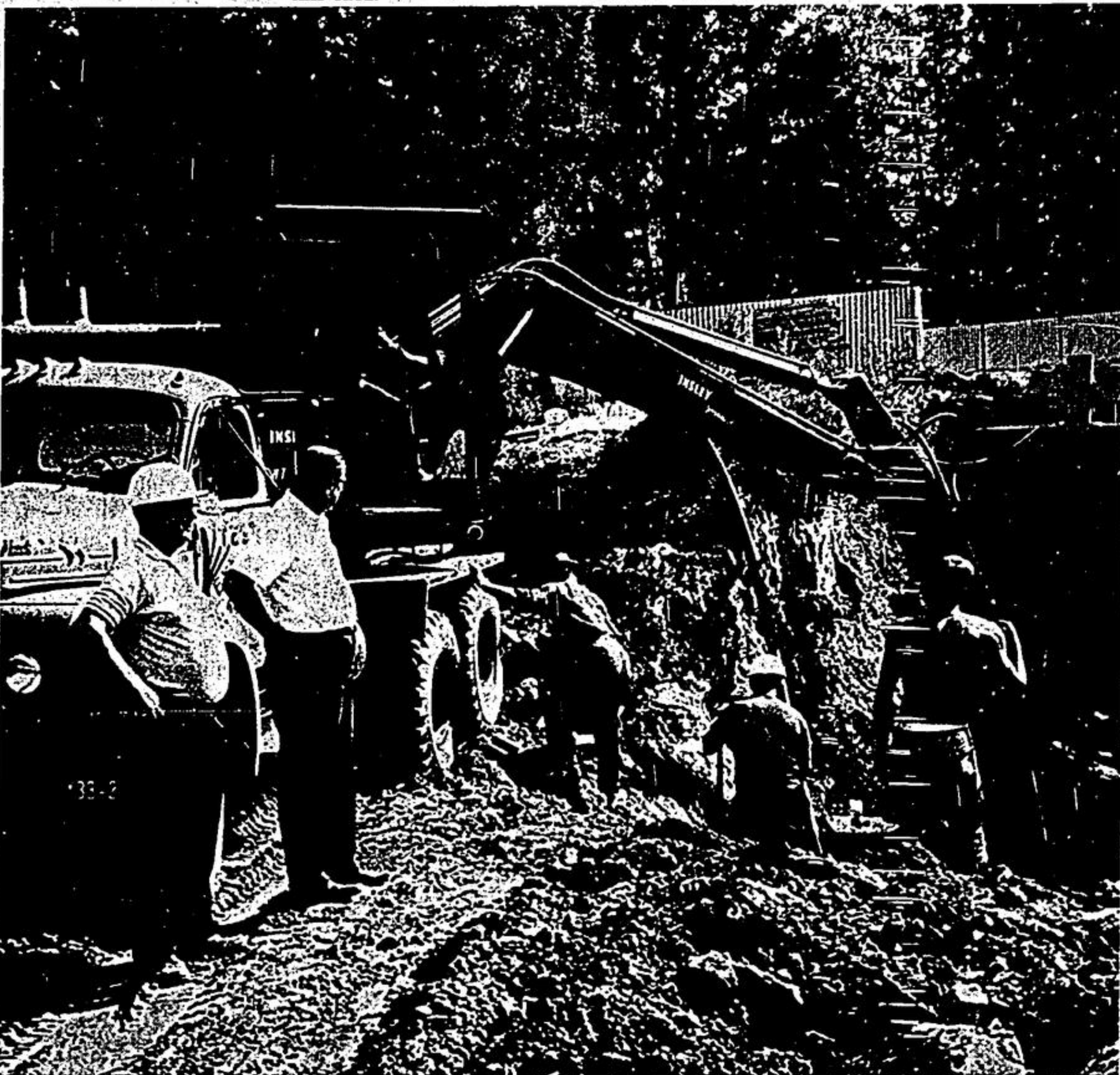
Contractor Ken Betz with hard hat is seen surveying the excavating of the new town water project on the town reservoir property. With him is Tommy Farr, chairman of the Stouffville PUC. Fred Castle is the shovel operator. Work on the project was begun last winter and will raise the water storage capacity to more than double the present figure. The new reservoir measures 110 ft. by 114 ft. and will cost approximately $45,000. Several new wells to feed this new storage will cost approximately $25,000. The work is expected to be completed this month. —Staff Photo
