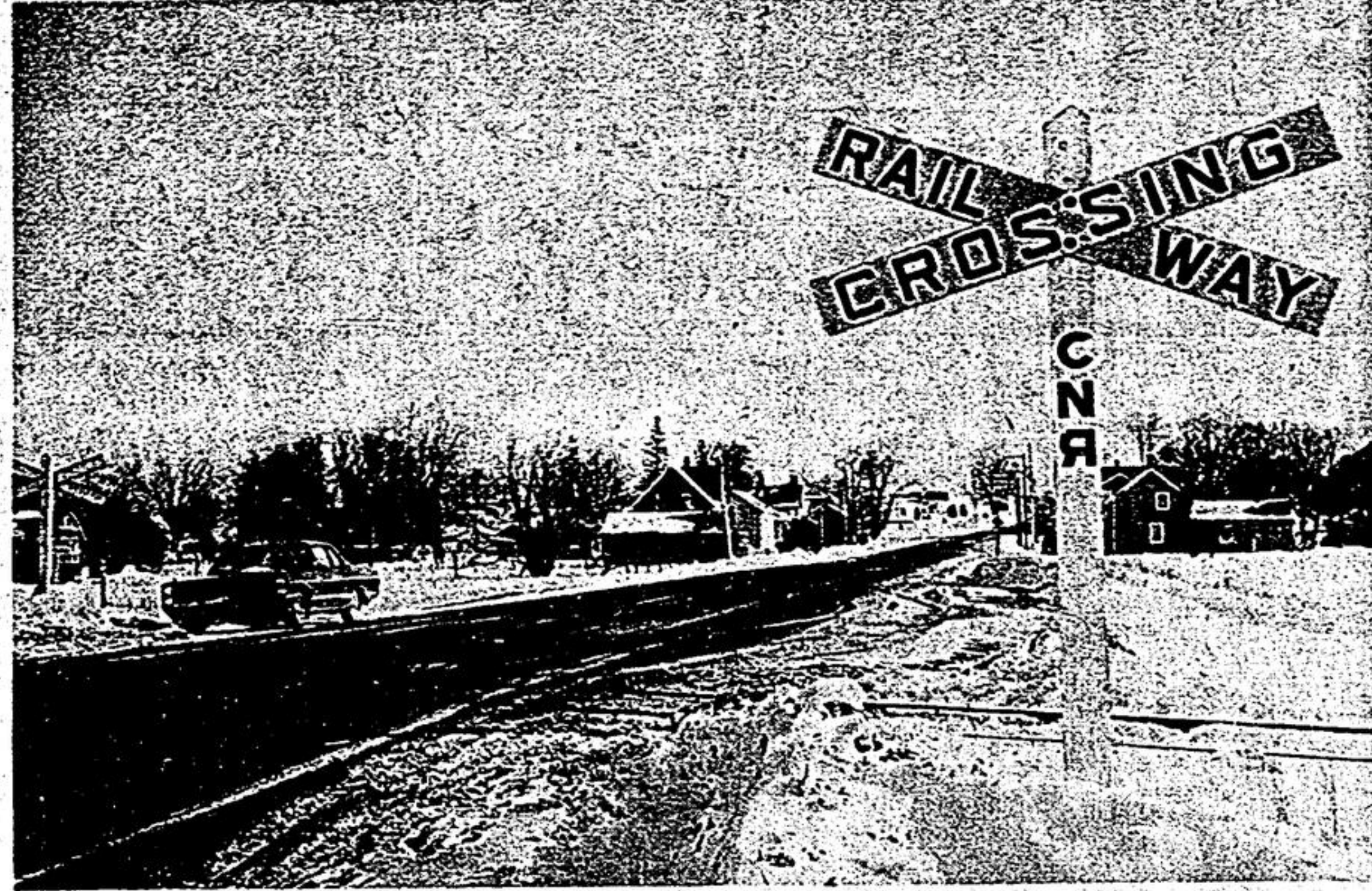
This crossing site on County Road 1A at Goodwood, is not protected by automatic signals. Uxbridge Township Council is agreeable to the installation of lights but the members feel that Ontario County should pay the full cost. — Staff Photo
