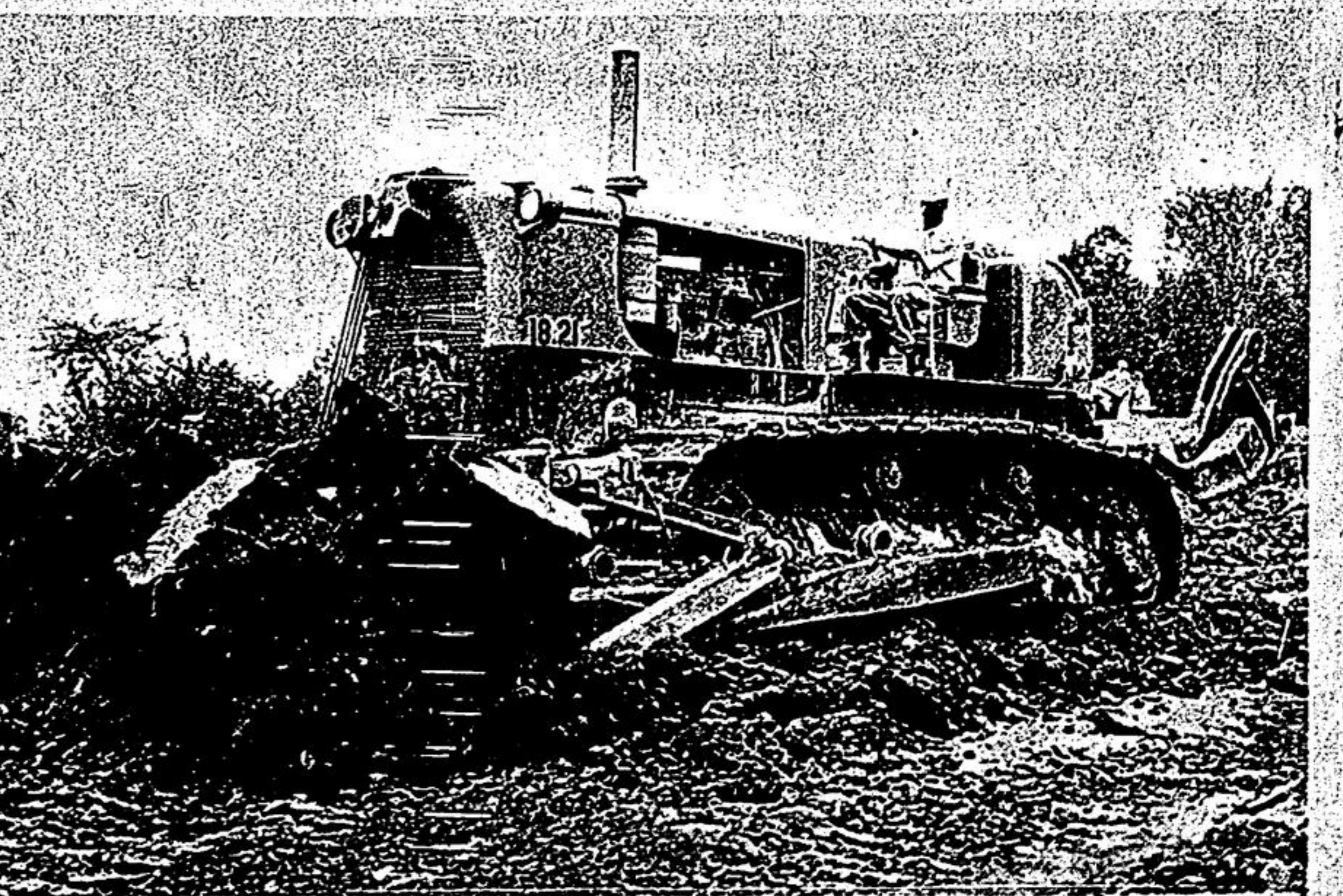
Begin Work on 140 Home Development in Stouffville's West End.
