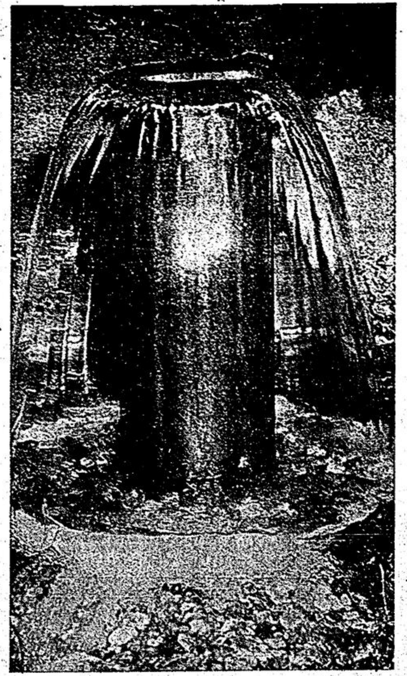
Although a water strike was made at a site north of Stouffville on the 9th conc. of Whitchurch Twp., P.U.C. Chairman Walter Atkinson feels that the supply is not sufficient to fill the town's need. Tests will be made to measure the flow. —Staff Photo.
