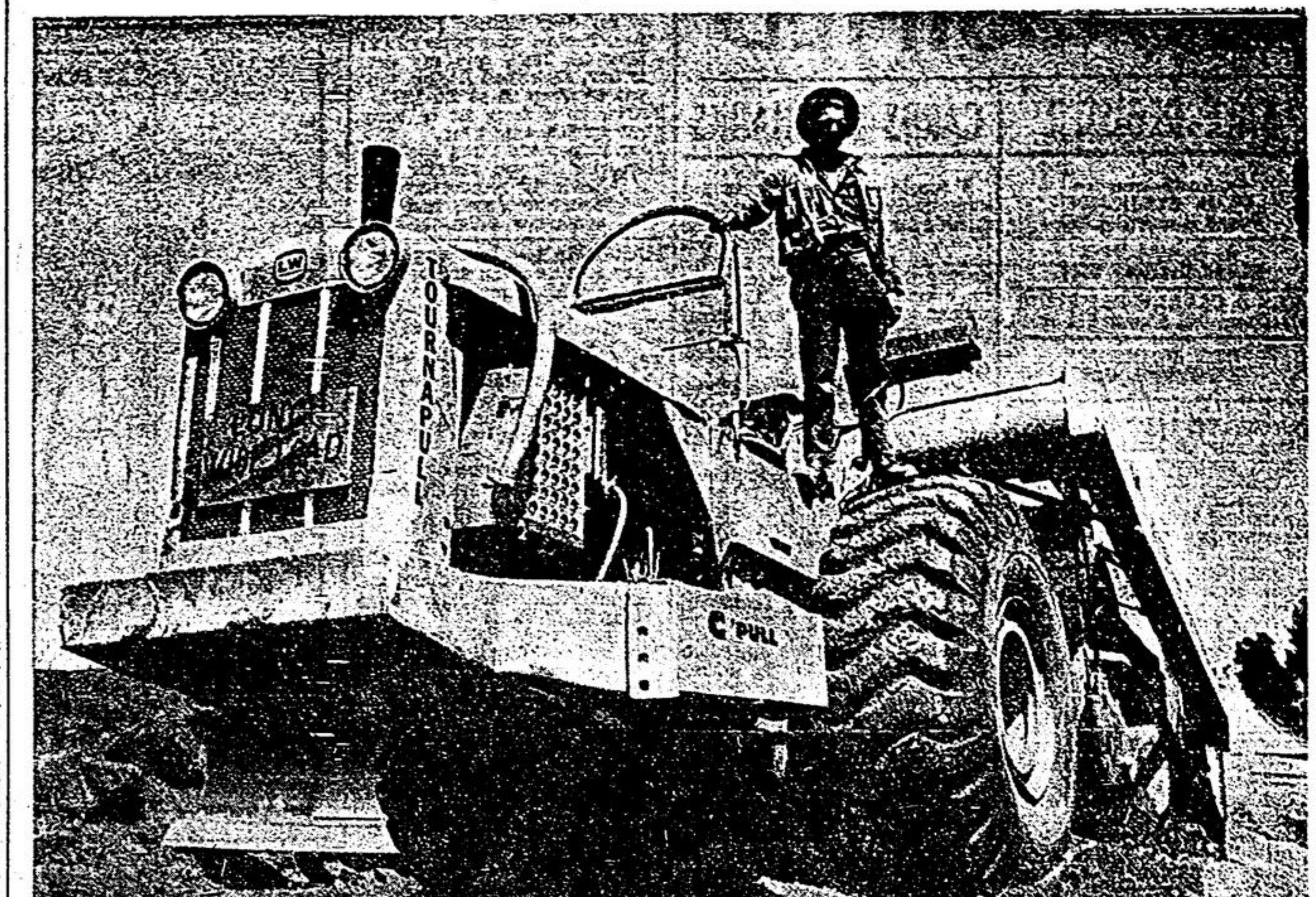
Vern Rose, a twenty-two year old operator of a 20-ton earth-moving machine, had a close call with death on Monday morning when his big diesel tractor flipped over on its nose. The accident occurred during construction on the County improvement road, east of Goodwood in Uxbridge Twp. The driver remained at the controls and escaped injury. The unit was not badly damaged. —Staff Photo
