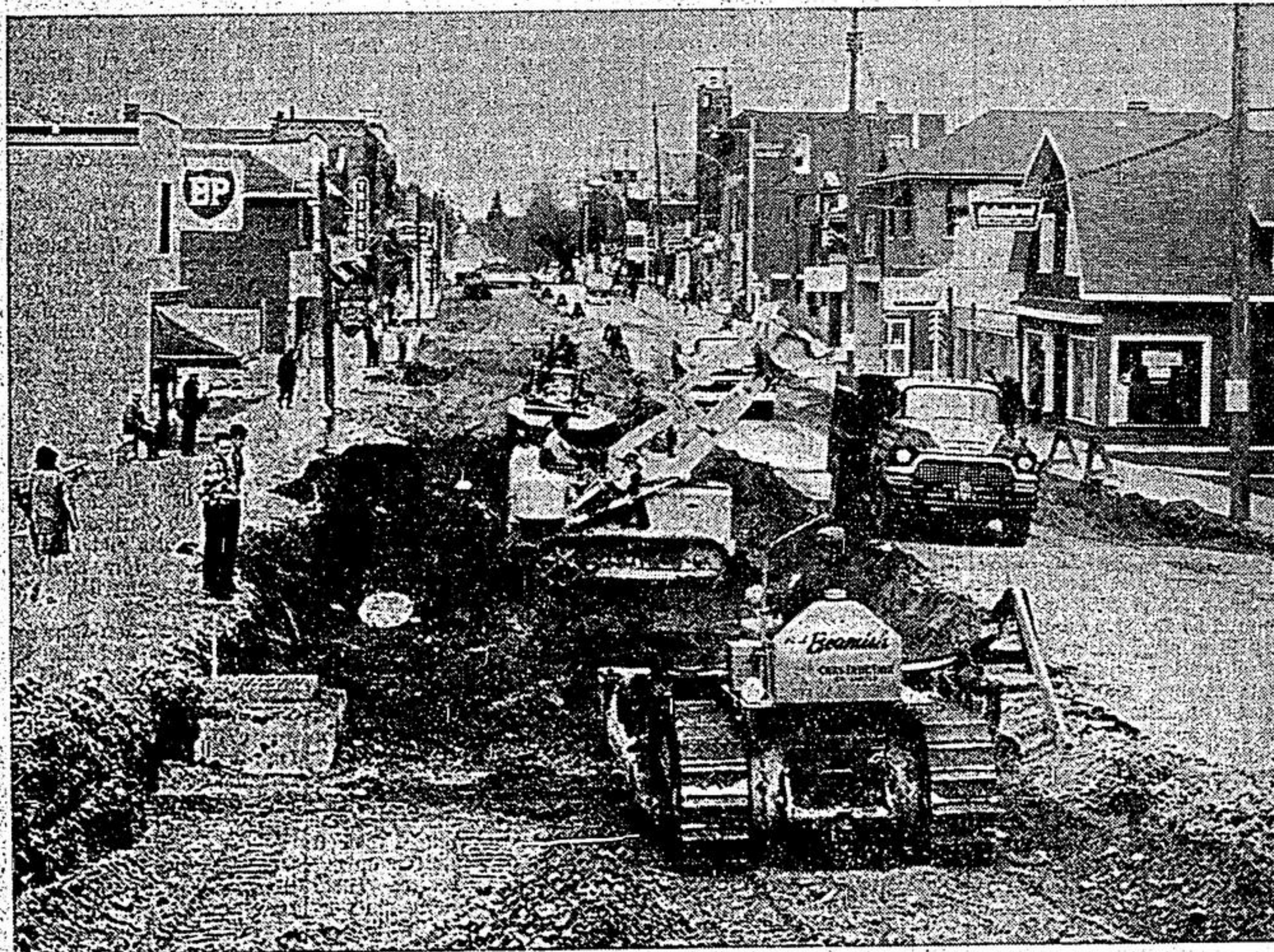
Main Street Pavement Construction
