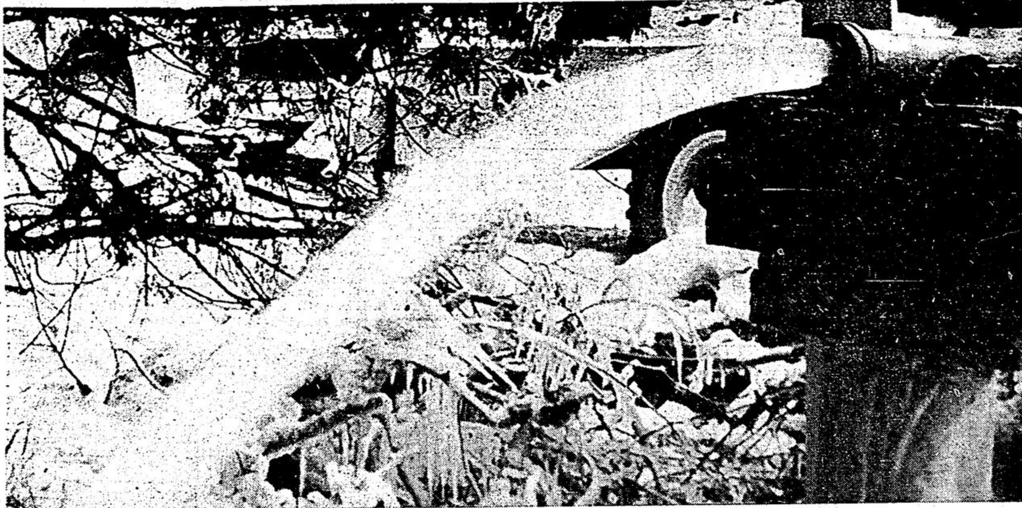
A new Stouffville well, producing an estimated 750 gallons of water per minute will provide for the future needs of town residents up to a population of 12,000 people. The strike was made on Thursday morning. A one-day test produced one million gallons of water in 24 hrs.—Staff Photo
