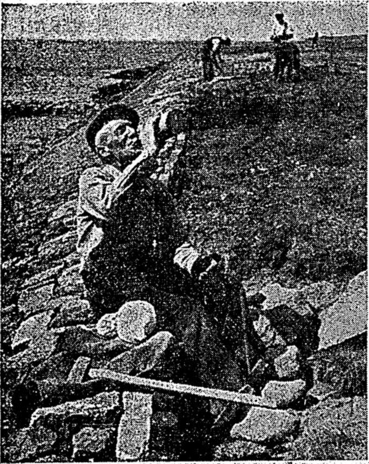
De Groet pauses for a drink after working on dike.
