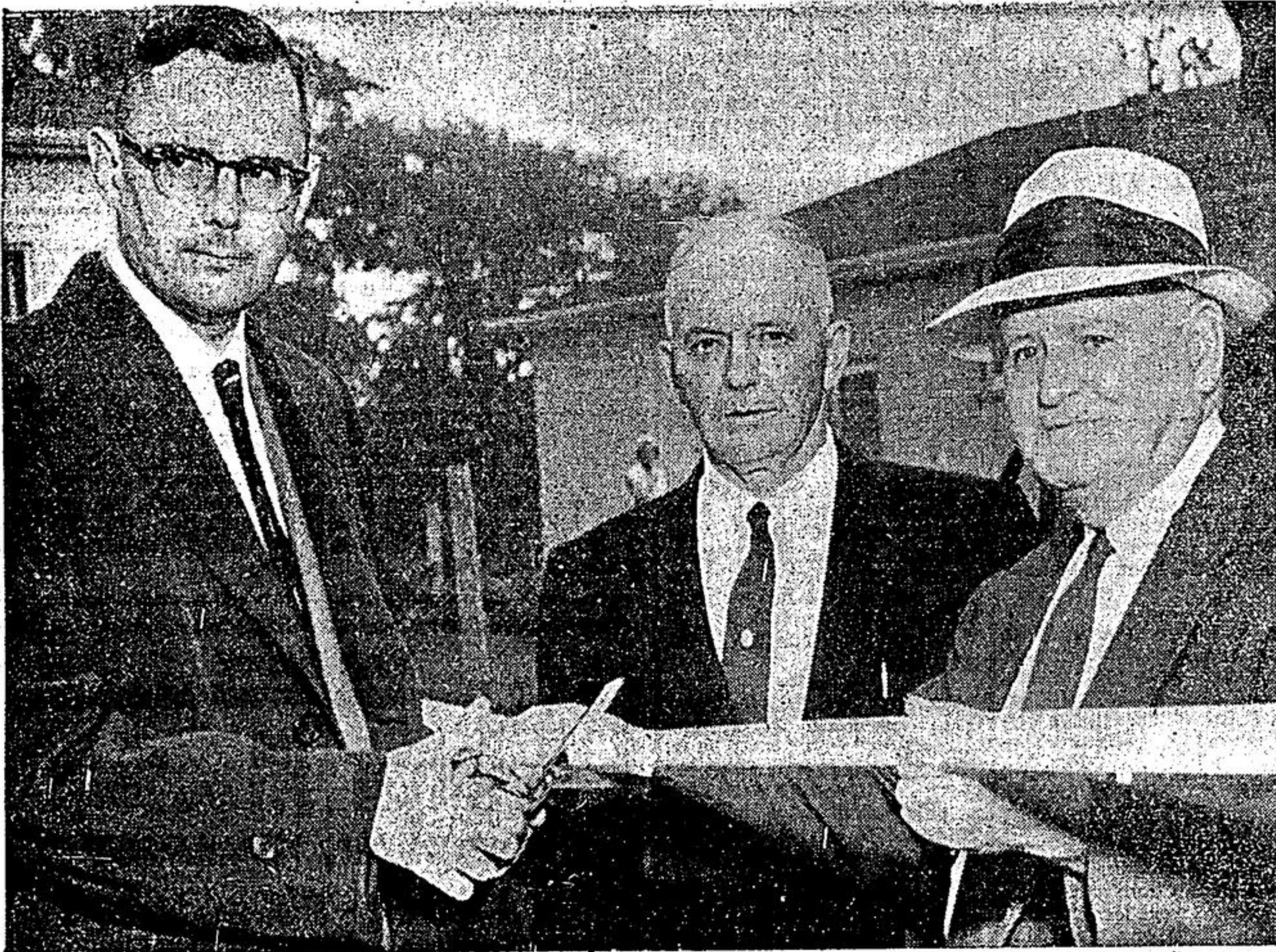
Open First Whitchurch Pavement
