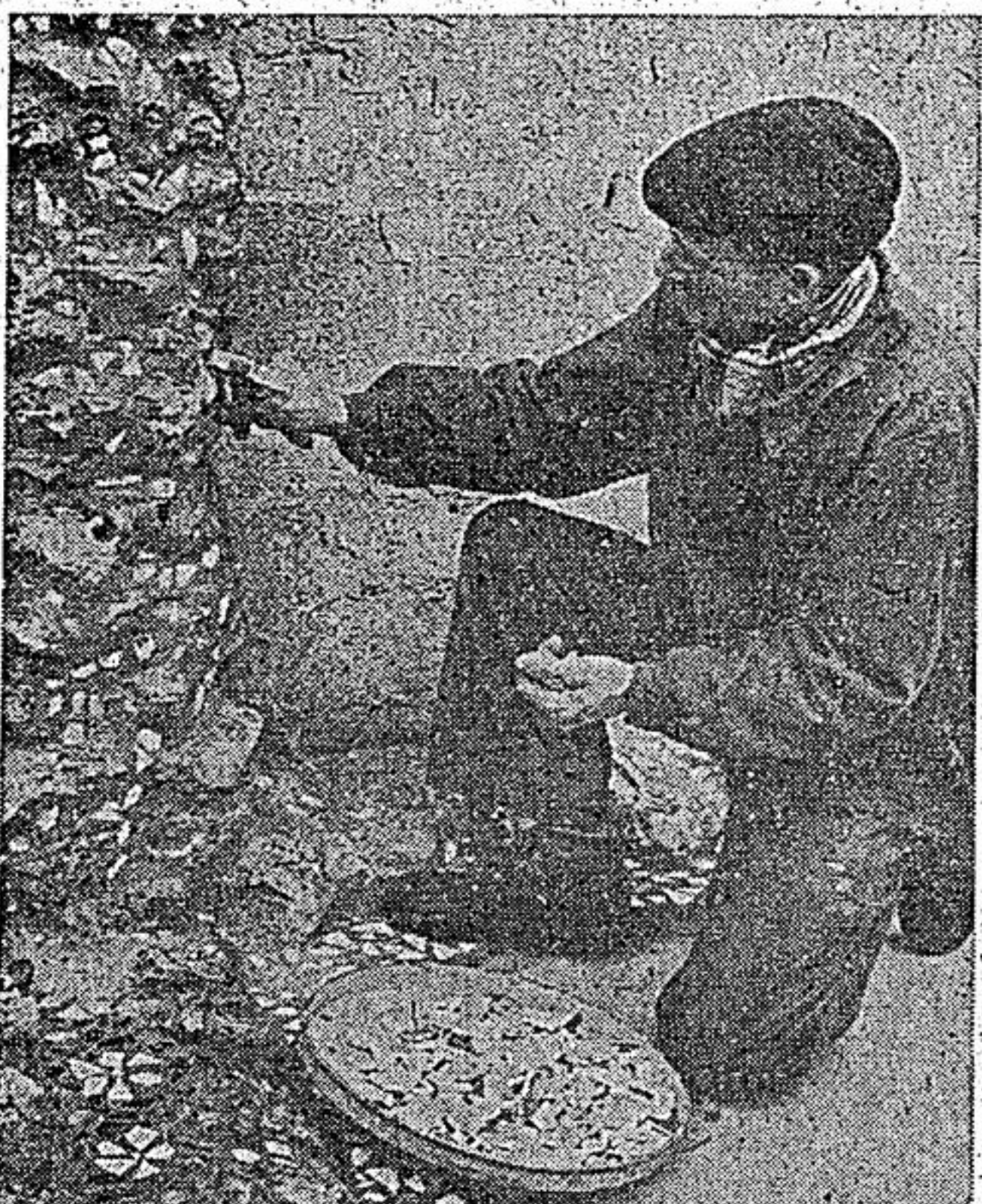
He's imbedding crockery pieces into section of house.
