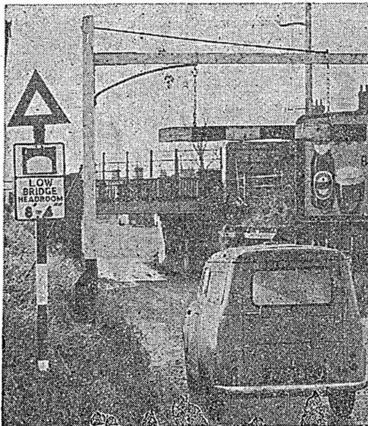
SHOCK ABSORBER —A road marker in front of a low bridge in Norfolk, England, prevents trucks from getting stuck. Trucks that can't get under the striped bar of the sign won't be able to clear bridge in background.
