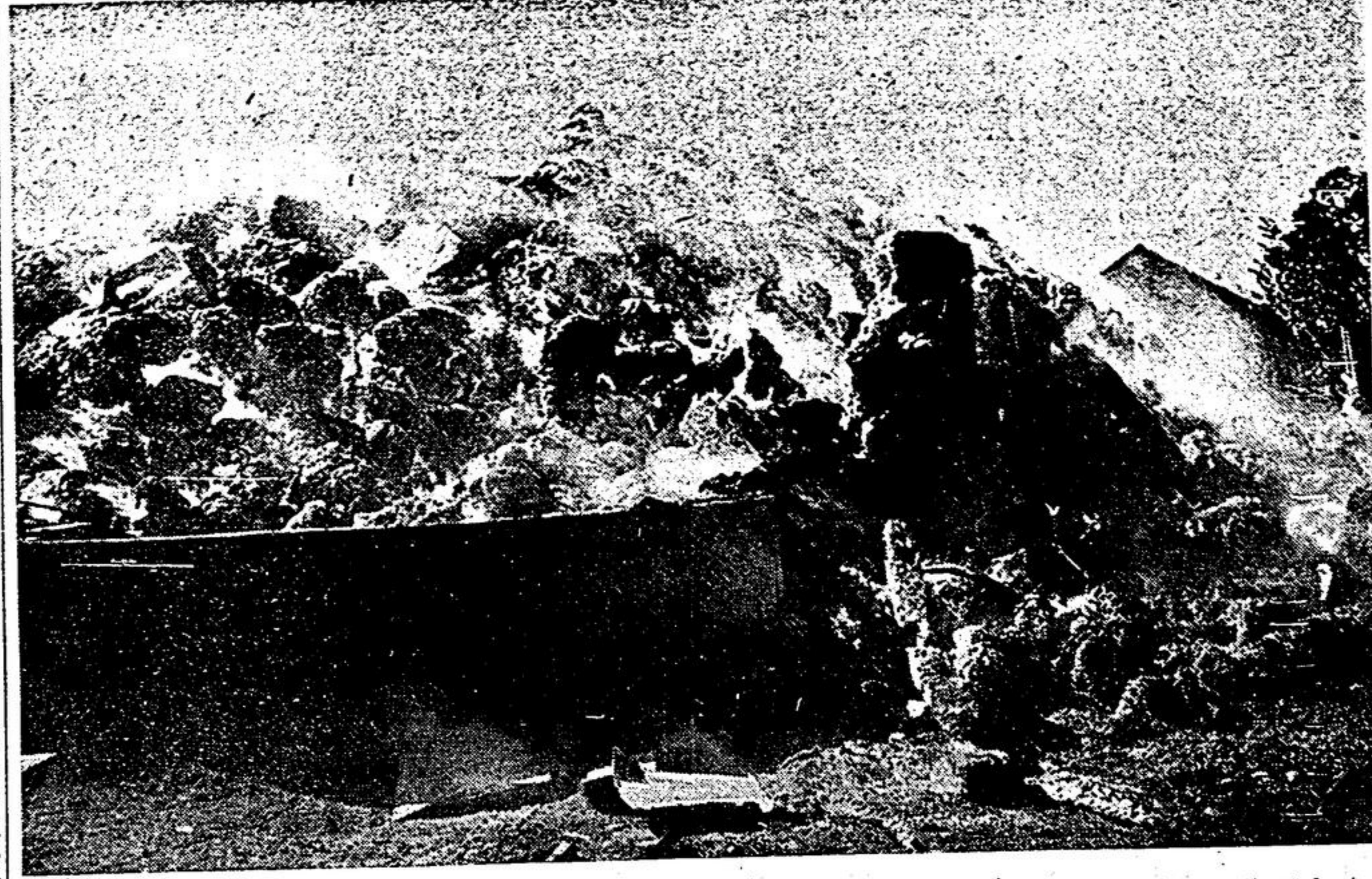
Smoldering ruins are all that remains of a large frame barn on the property of Mr. John Dowling, 8th concession of Pickering near Claremont. The fire broke out on Thursday morning of last week and in a matter of minutes, the structure was levelled. The loss has been estimated at $15,000. —Jim Thomas
