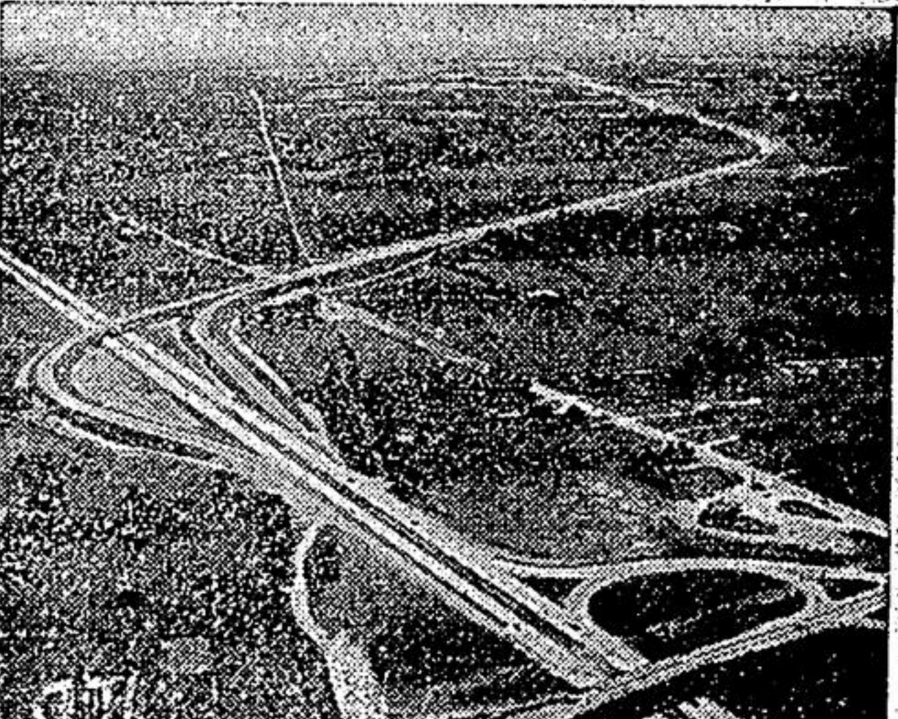
Eastern Terminal portion of the Toronto Bypass with extended view of its curving approach over Highway No. 2, and its continuation as Highway 401 easterly (bottom of picture) to Oshawa, Bowmanville and Newcastle. This air photo shows how Ont. Dept. of Highways planning experts provided for Toronto Bypass direct entrance to and egress from Toronto-Oshawa four-lane Highway. That is, traffic does not use cloverleaf except for connection with Lansing Cutoff Road.
