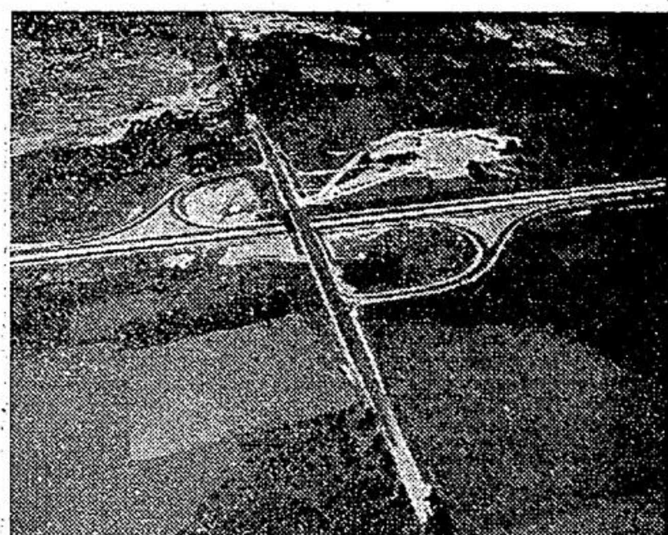
Little's Road Overpass of newly opened eastern section of the Toronto Bypass and 2-level traffic interchange. This air photo shows how the Ont. Dept. of Highways is planning to take care of traffic increases in this area when before long, community development will follow the growth pattern in Metropolitan Toronto which has been greatly encouraged by the now completed Toronto Bypass or Interceptor portion of Highway 401, 21 miles long, and some five miles of rebuilt Highway 27 which link it with the Queen Elizabeth Way just west of the Humber River.
