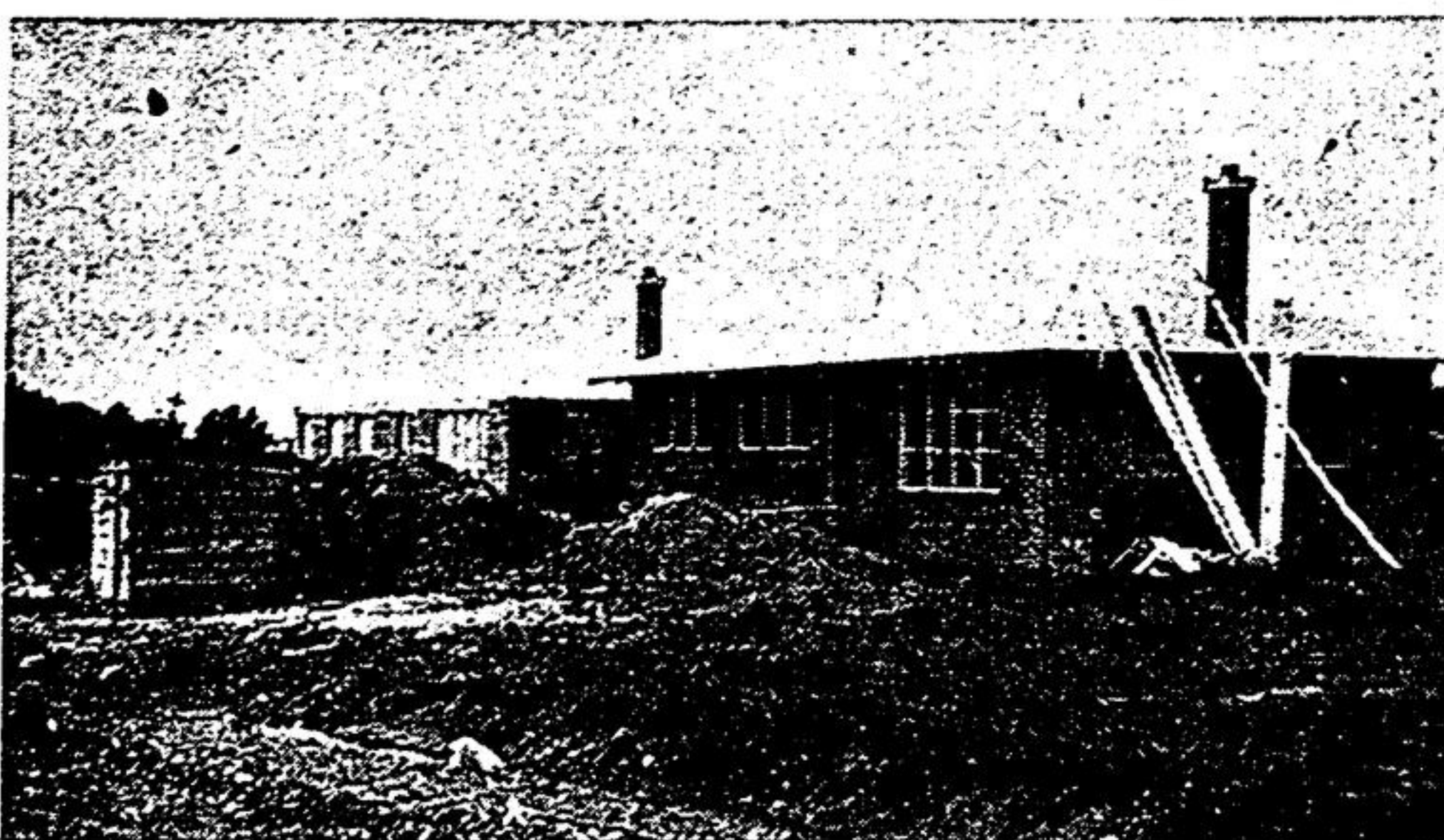
Some of the N.H.A. homes being erected on the Hawtin sub-division are shown here in process of construction. Excavations for four more homes have also been made on the Timbers sub-division. S. M. Sinclair, local real estate man, is in charge of the Hawtin development.
