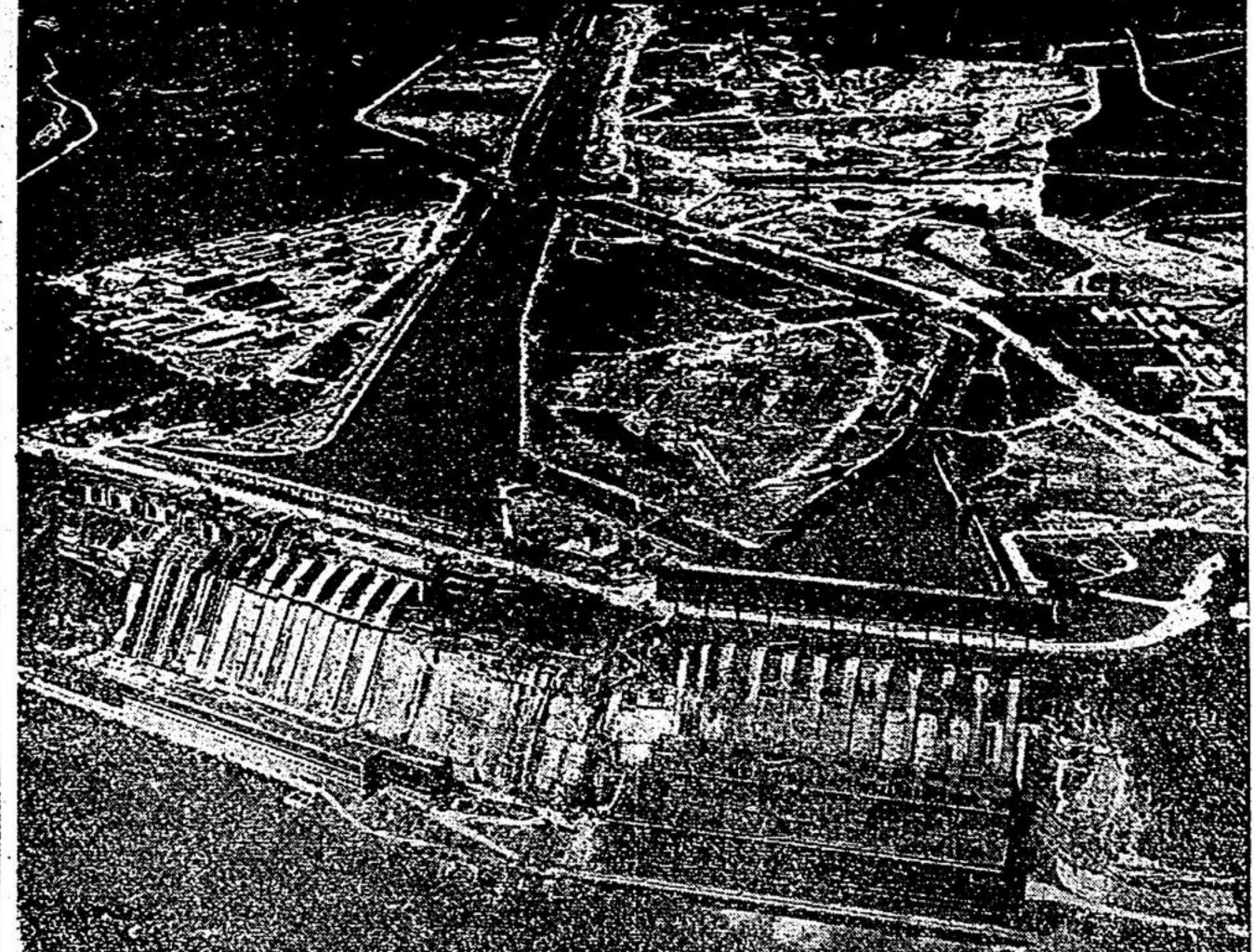
CUT —Pride of Ontario Hydro Here, where three-and-a-half years ago there were only the bare and ancient rocks of the 300-foot cliffs of the Lower Niagara Gorge, Ontario Hydro engineers and workmen have created the modern giant of the 1,525,000 horsepower Sir Adam Beck-
