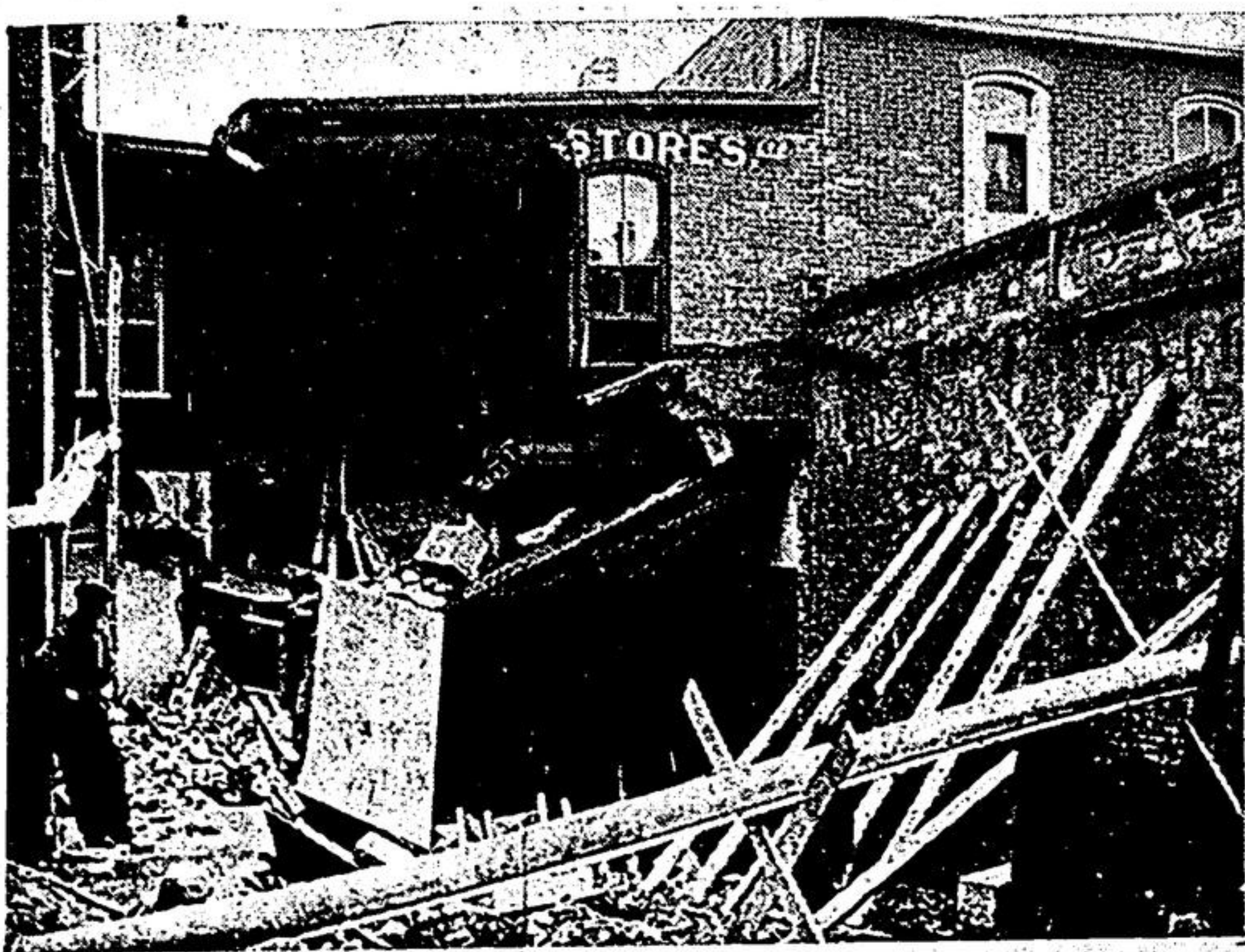
Employees of the Russ Far Construction Co. luckily escaped serious injury on Tuesday afternoon when the rear section of the Dominion
