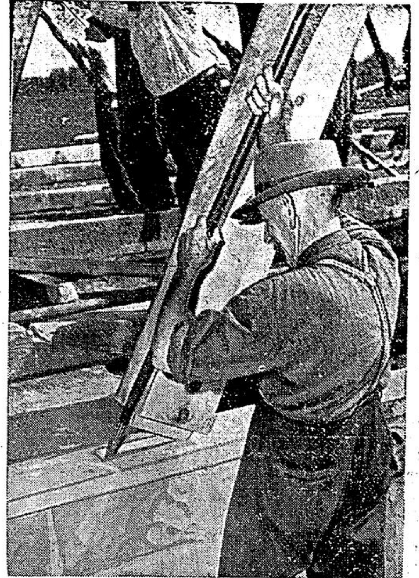
Easing a main post into its mortise is not a simple task for John Scott, Stouffville, once Markham Fair President.
